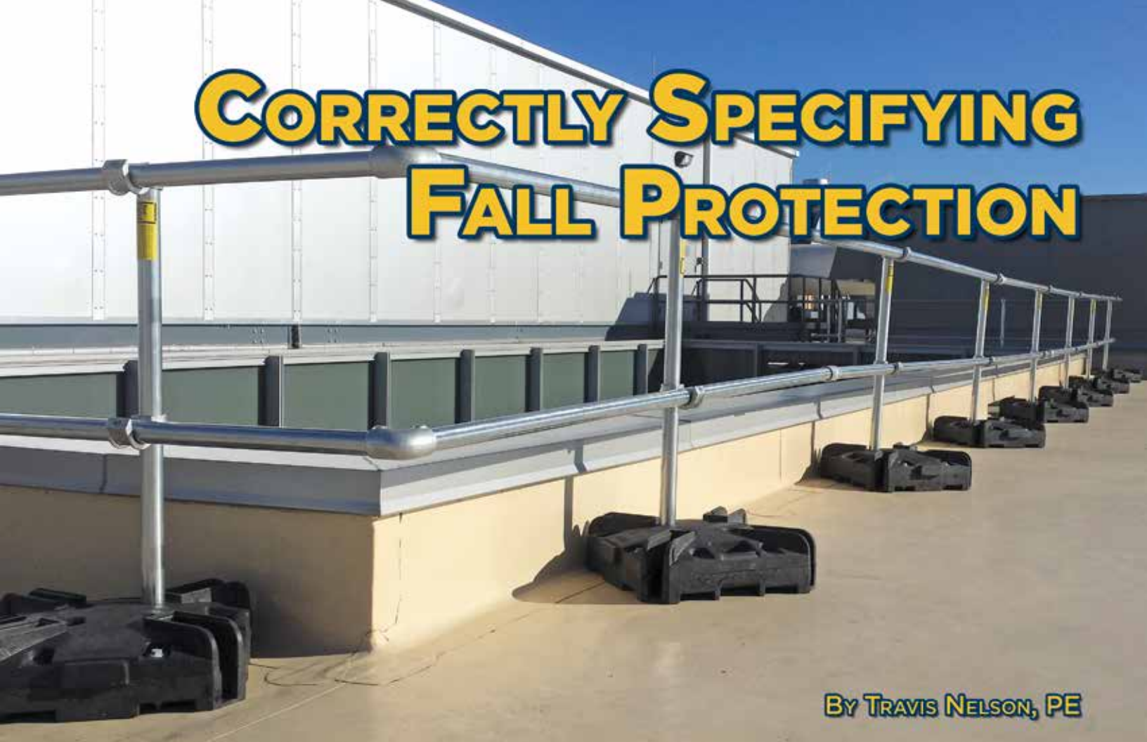
Figure 1 – Ballasted guardrail system.
