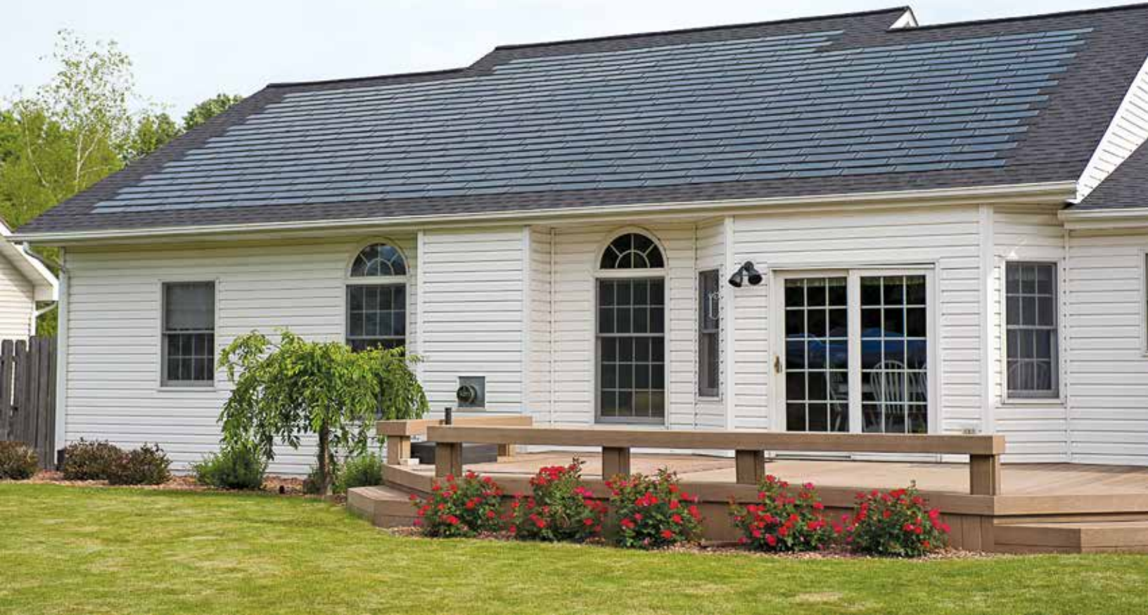
Photo 1 – Home sporting Dow’s Powerhouse Solar Shingle system.
