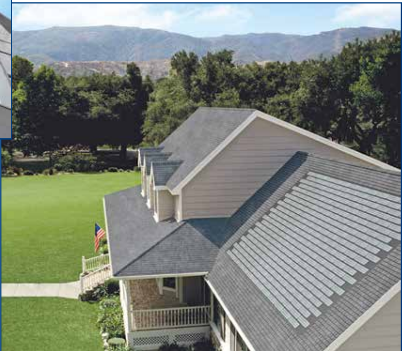
Photo 4 – Building-integrated PVs are less obtrusive and more visually pleasing. Dow’s Powerhouse Solar Shingle was named one of the “50 Best Inventions of 2009” by Time magazine.
