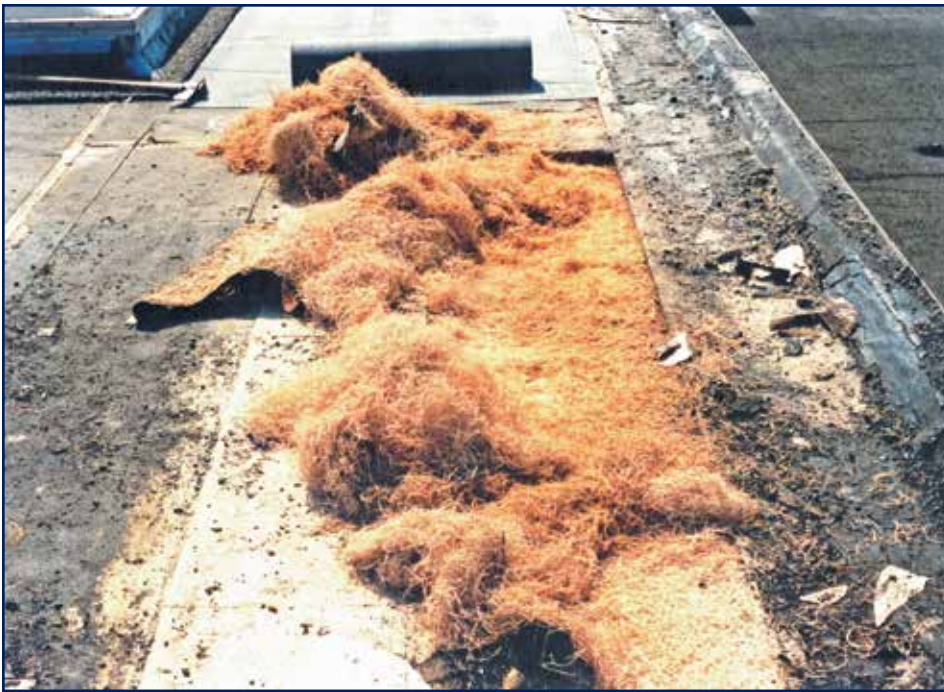
Figure 9 – Manufacturing flaws (although infrequent) can include improperly blended ingredients.
