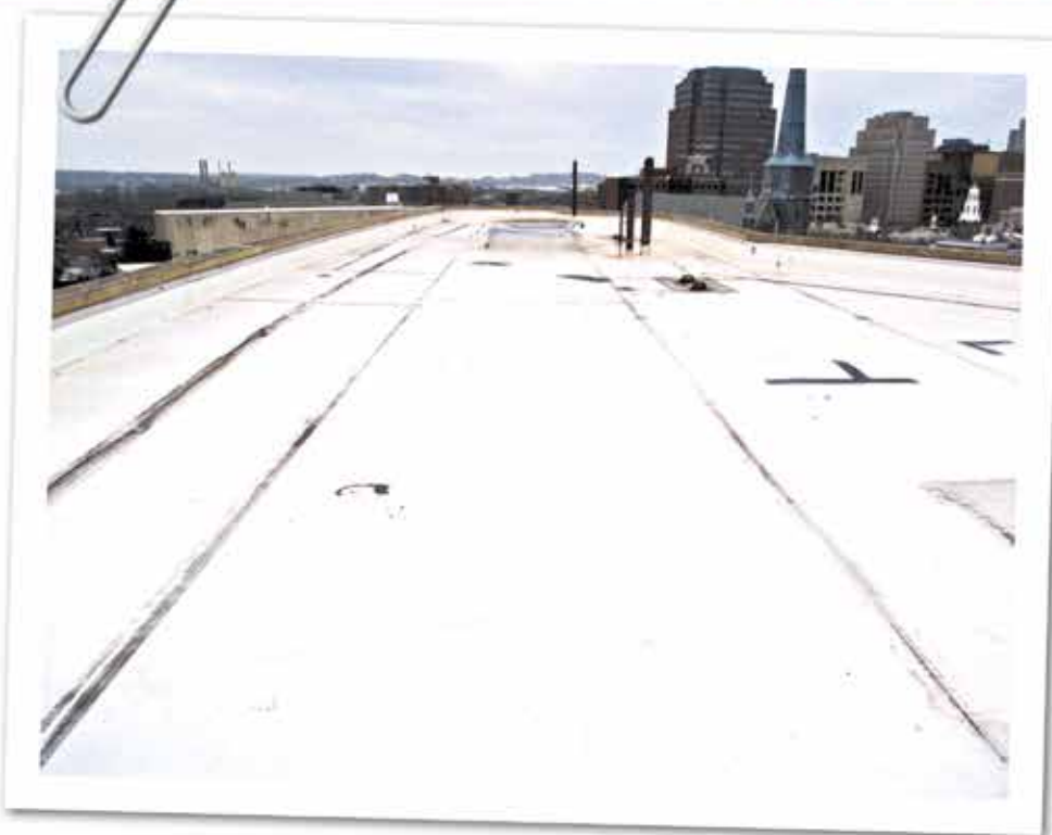
Figure 2 – Overview of roof.
