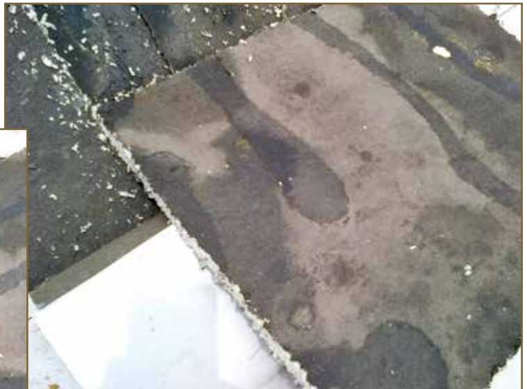
Photo 9 – Moisture between the layers of boards.
