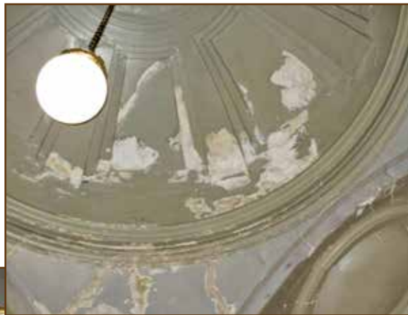
Figures 1A and 1B – Plaster damage occurred after insulation was installed above the domes.
