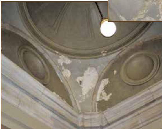
Figures 1A and 1B – Plaster damage occurred after insulation was installed above the domes.
