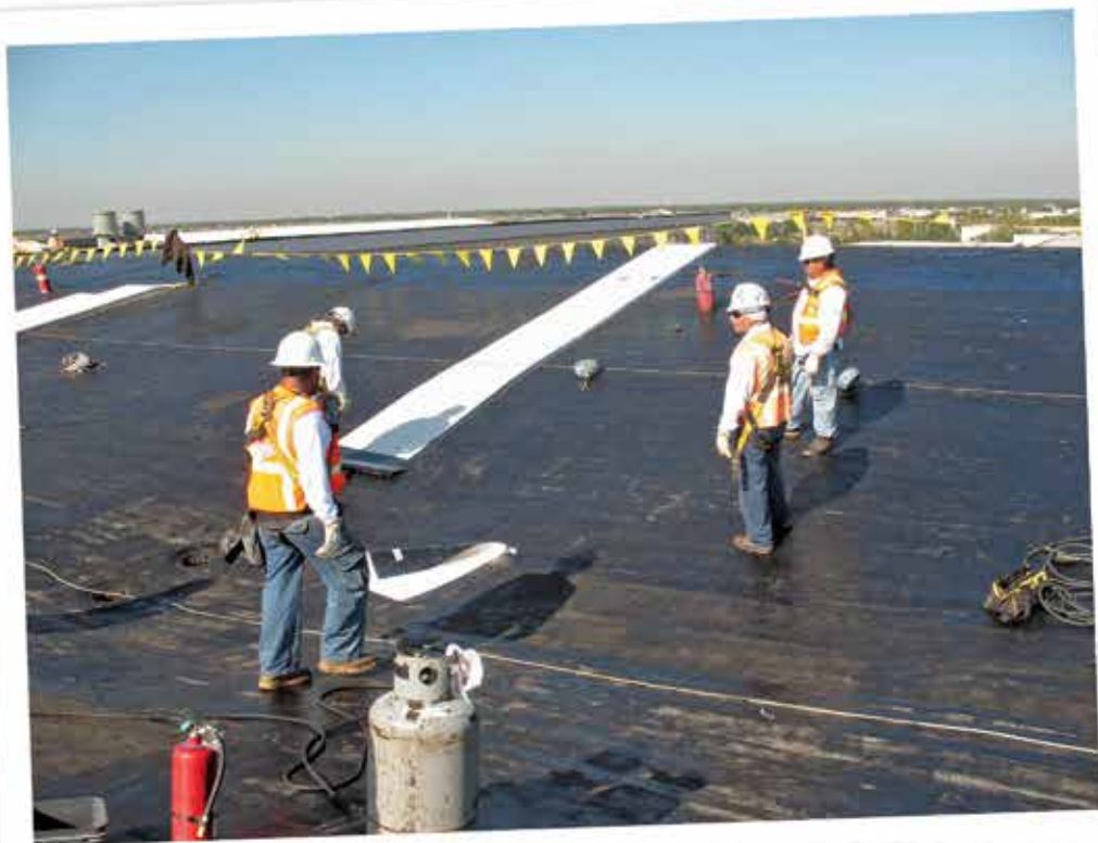
Site visit. Photo courtesy of Building Solutions, LLC.
