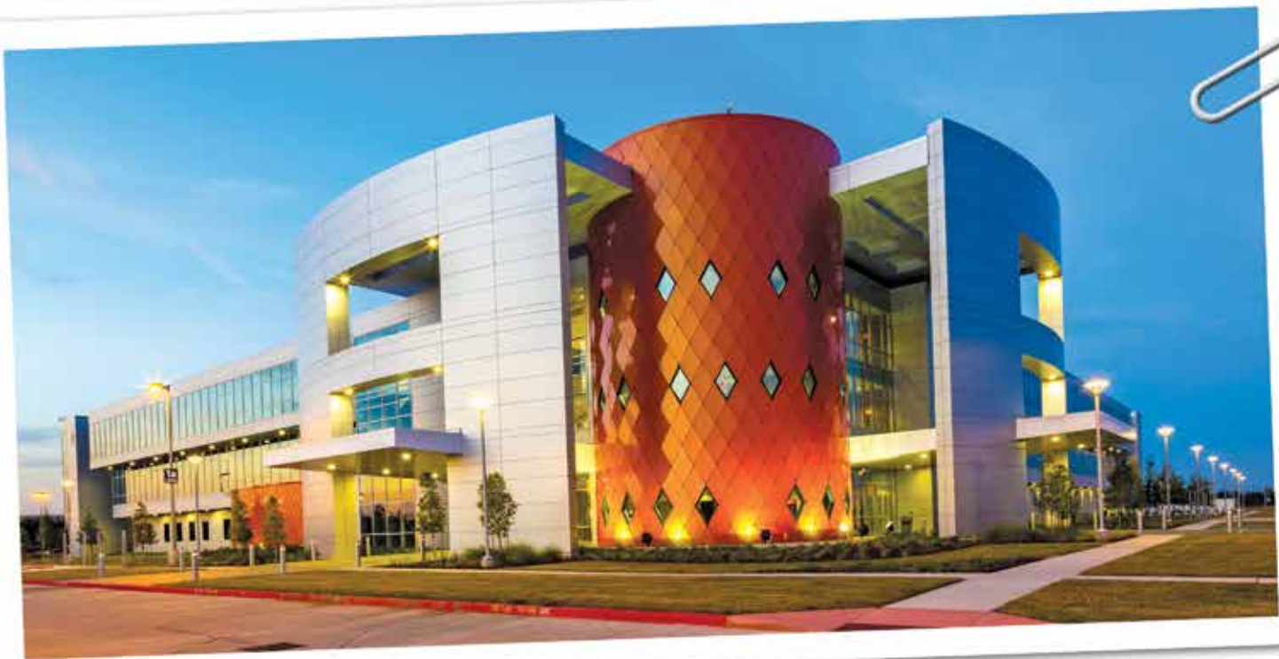
Photo courtesy of Bay-IBI Group Architects and Slyworks Photography.
