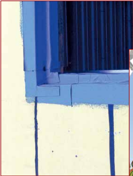
Figure 7 – When using a shingled series of straight and flexible flashing or both to waterproof the rough opening, it is easy to underestimate the impact several layers of thick membranes have on the distance between corners of the rough opening.
