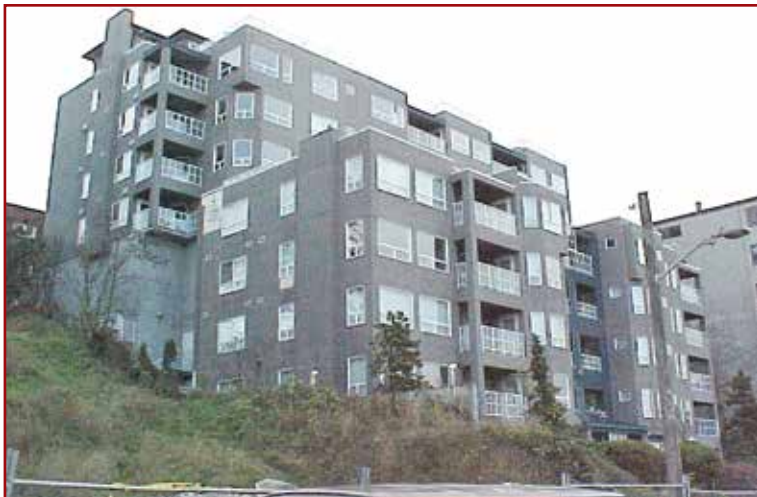
Figure 2 – Energy-efficient walls that incorporate windows constructed with multi-layered, gas-filled, insulated glass with low-e films and thermally efficient window frames make it easy to justify an increased footprint and a higher window-to-wall ratio.
