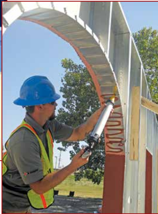
Figure 7 – When using a shingled series of straight and flexible flashing or both to waterproof the rough opening, it is easy to underestimate the impact several layers of thick membranes have on the distance between corners of the rough opening.
