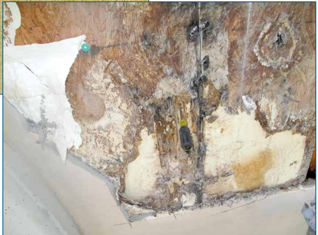
Figures 3 and 4 – Fractures in stucco allowed capillary suction across wall assembly, resulting in deterioration of the wall sheathing and framing.
