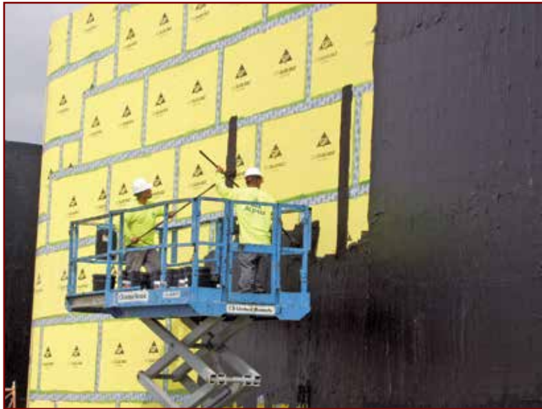
Photo 1 – Application of emulsion dampproofing.
