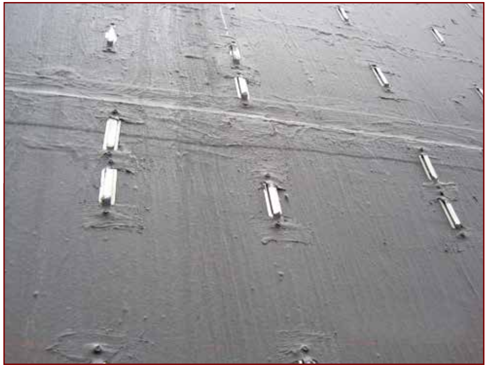
Photo 6 – Sealant applied over fastener heads securing brick ties.
