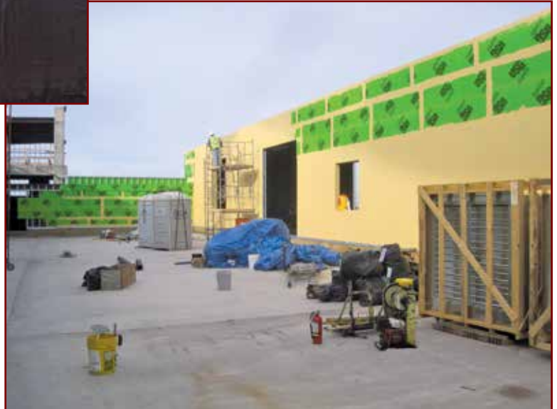
Photo 2 – Application of liquid-applied WRB.
