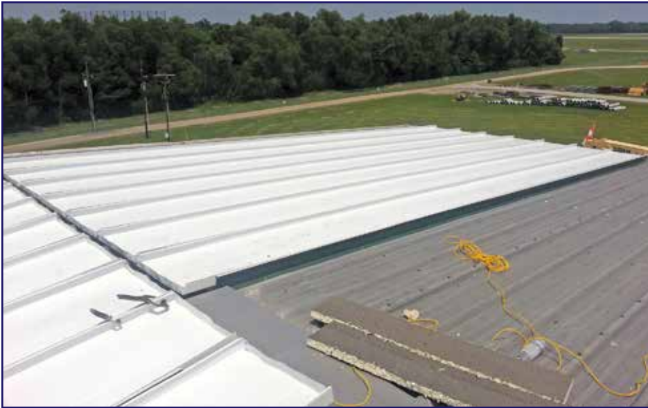
Figure 6 – Installation of the 24-gauge Galvalume symmetrical panels.
