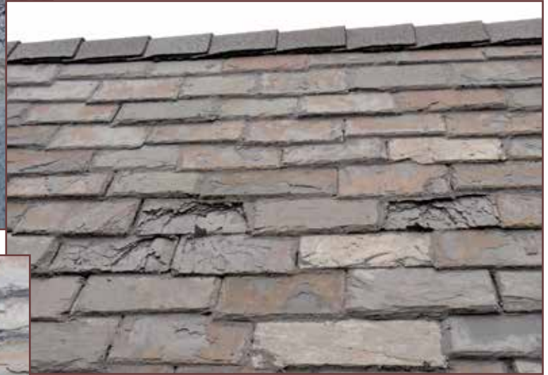
Figure 6 – Overview of freeze/thaw-damaged slate after grouting.
