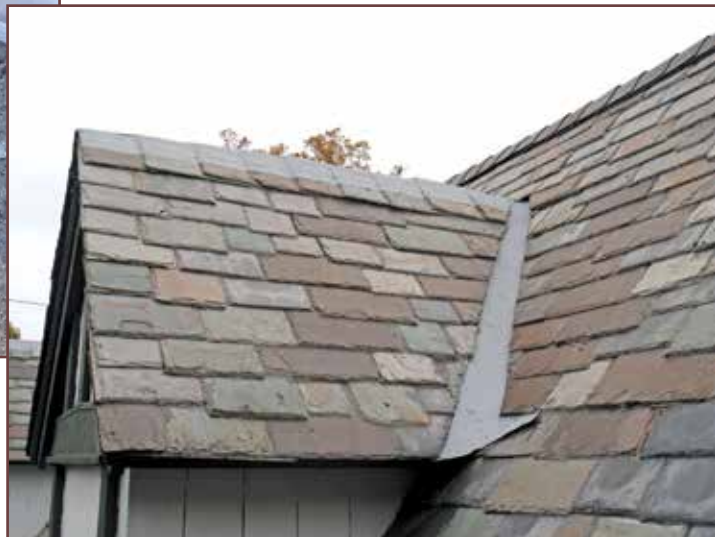
Figure 4 – Installation of reinforced liquid flashings.
