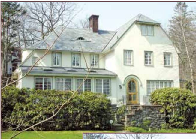
Figure 12 – Overview prior to slate grouting (photo courtesy of SlateSavers).
