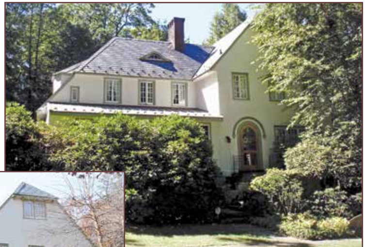
Figure 14 – Overview eight years after grouting.
