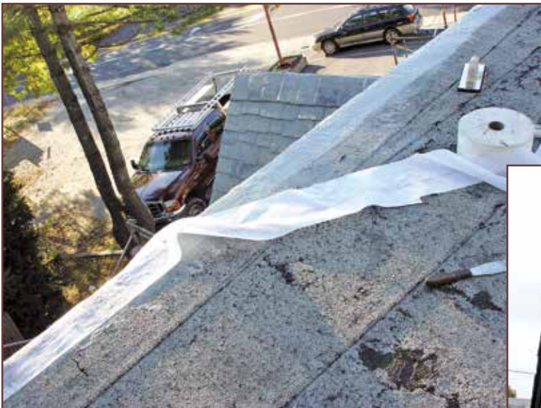
Figure 3 – Installation of reinforced liquid flashings (photo courtesy of SlateSavers).
