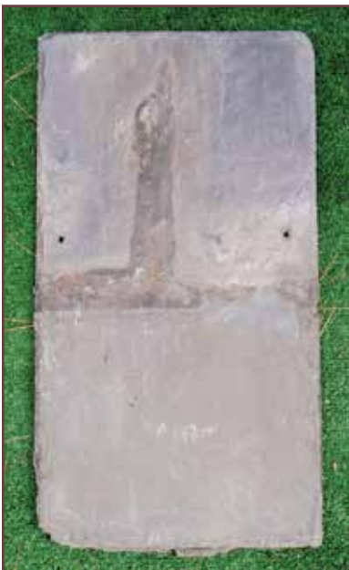
Figure 8 – Depth of penetration of grout injection.
