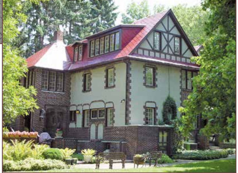
Figure 17 – Overview after tile grouting (photo courtesy of SlateSavers).
