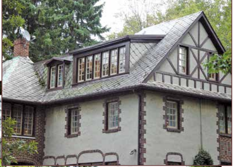
Figure 16 – Overview before tile grouting (photo courtesy of SlateSavers).
