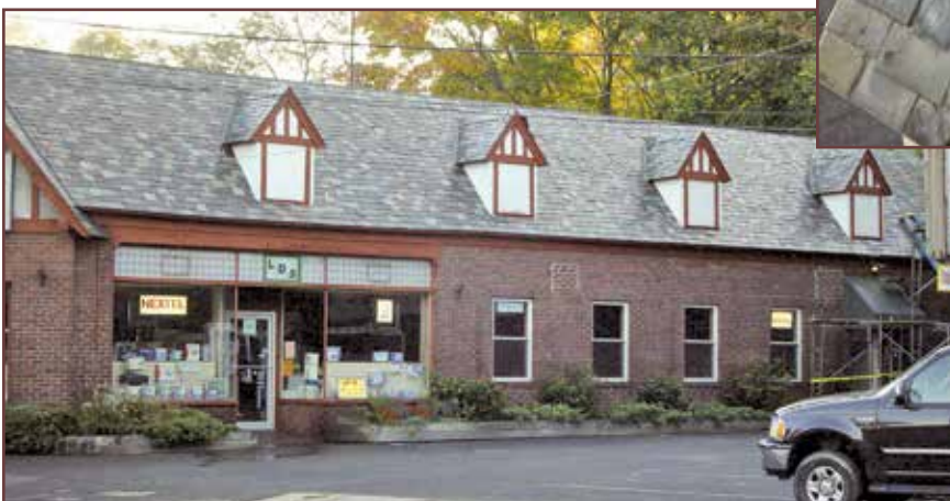
Figure 1 – Overview of varied-color slate roof.
