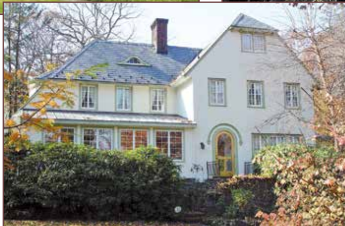
Figure 13 – Overview two years after grouting (photo courtesy of SlateSavers).
