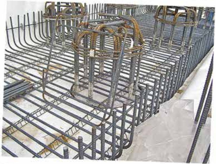
Photo 2 – Steel reinforcing in piers.
