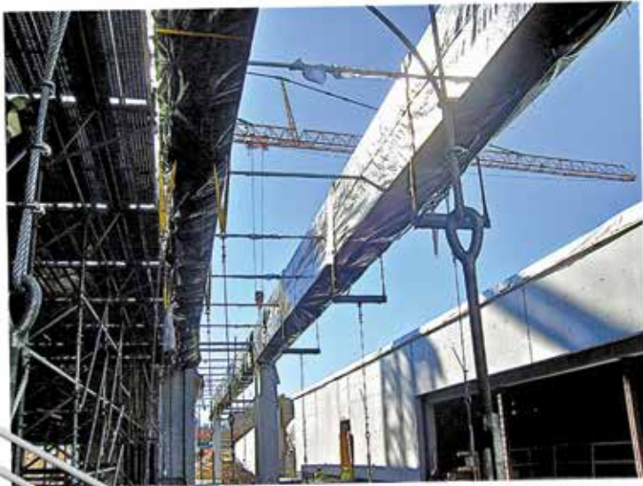
Photo 7 – Douglas-fir “glue-lam” beams.
