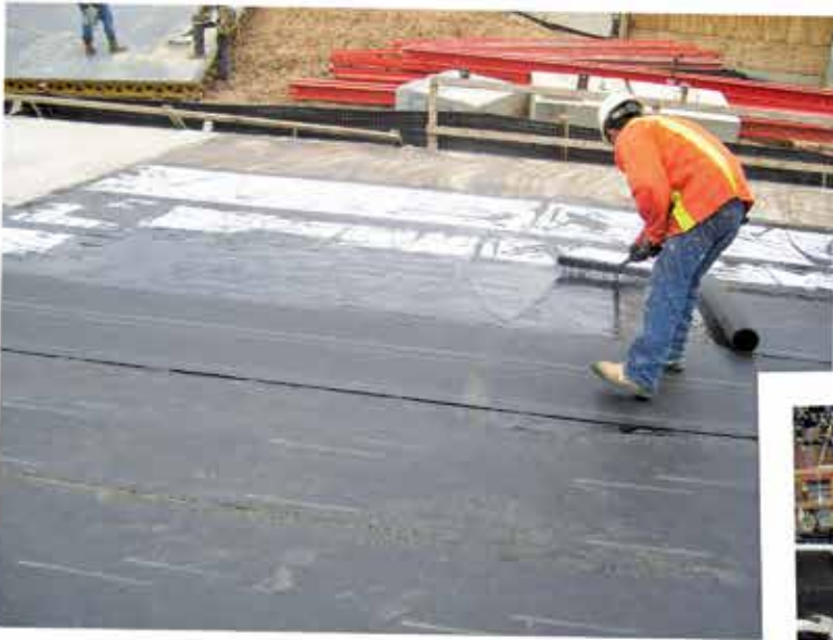
Photo 4 – Modified asphalt with polyester reinforcement.
