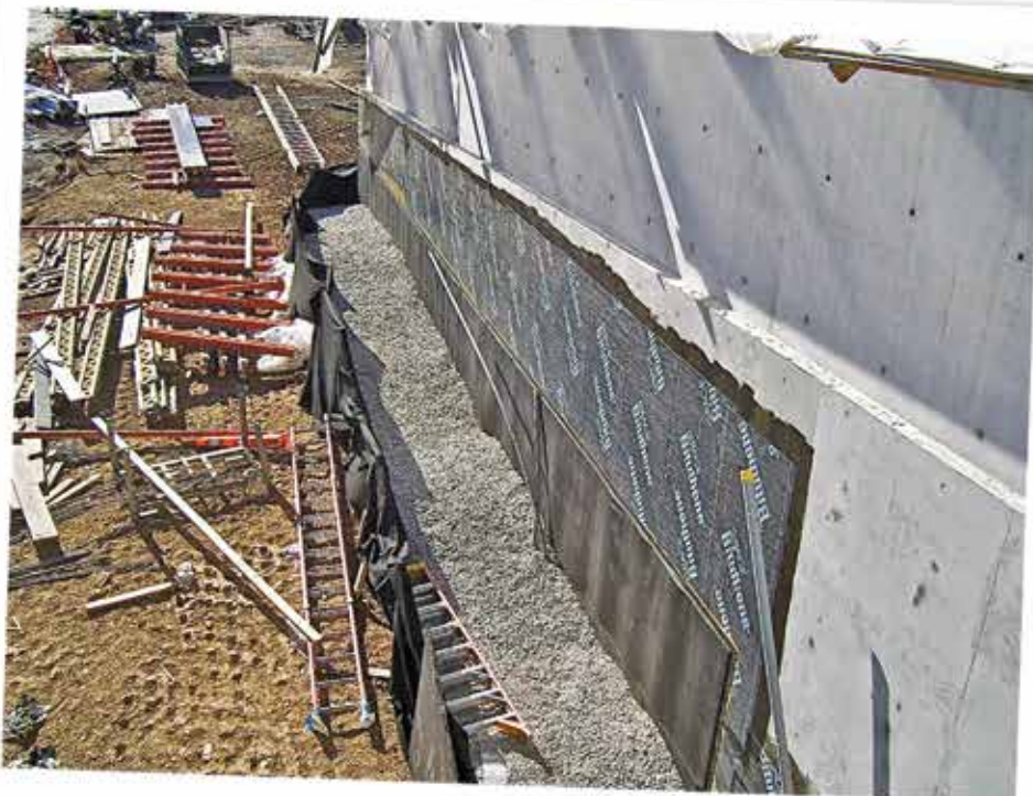
Photo 3 – Self-adhering waterproofing membrane.
