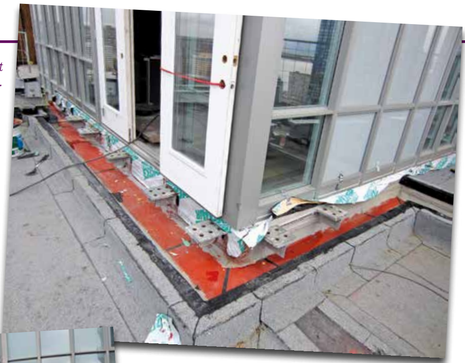
Photo 6 – Completed installation of the east tower expansion joint.
