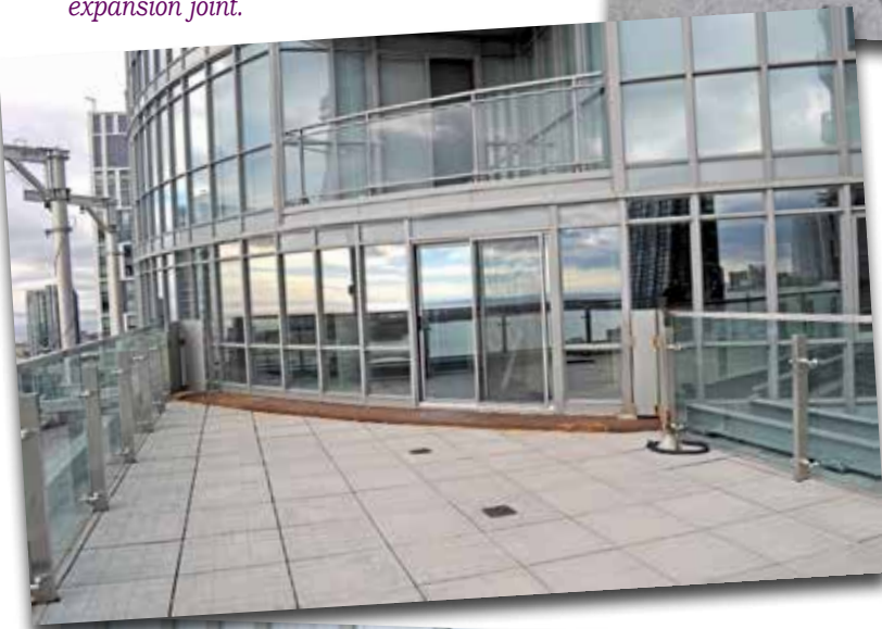
Photo 7 – Finished private rooftop patio looking at the west tower expansion joint.
