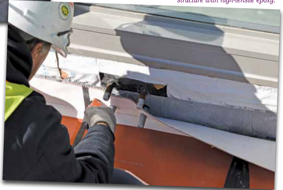
Photo 2 – The expansion joint is adhered to the structure with high-tensile epoxy.
