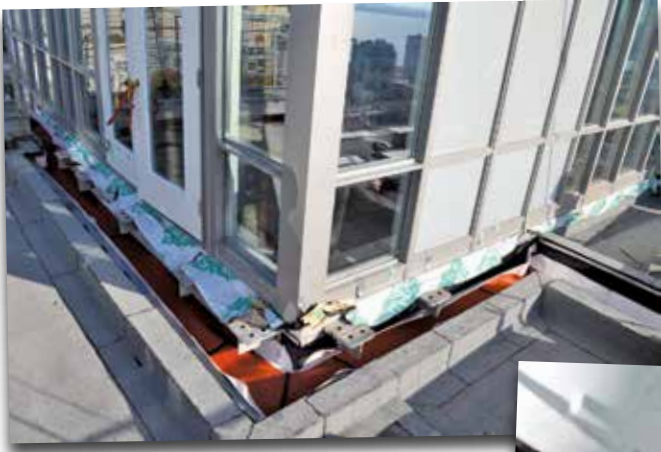
Photo 1 – The east tower joint is being dry-fitted.
