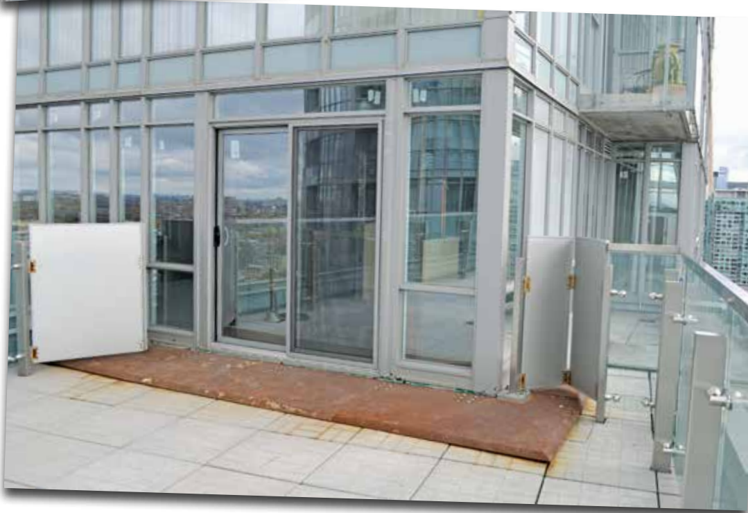
Photo 8 – Finished private rooftop patio (facing the east tower expansion joint).
