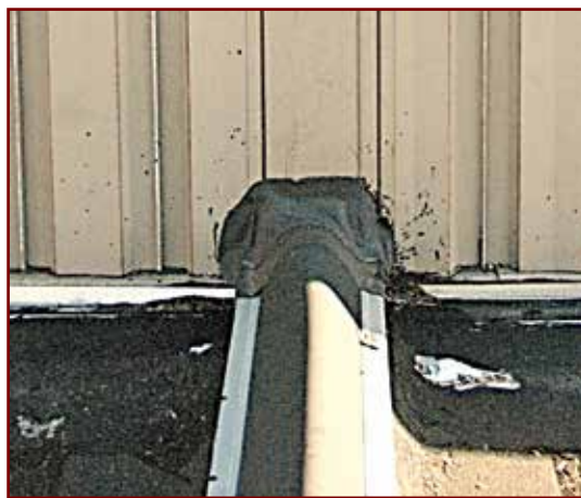
Figure 2 – Field condition of a seven-way primary transition with combined changes.
