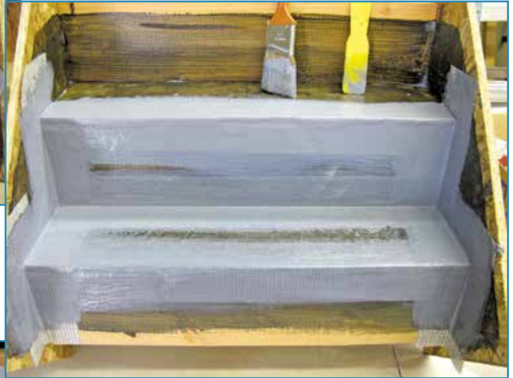
Photo 17 – Lay fabric into a coat of acrylic, typically working from bottom up. Smooth with overcoat.
