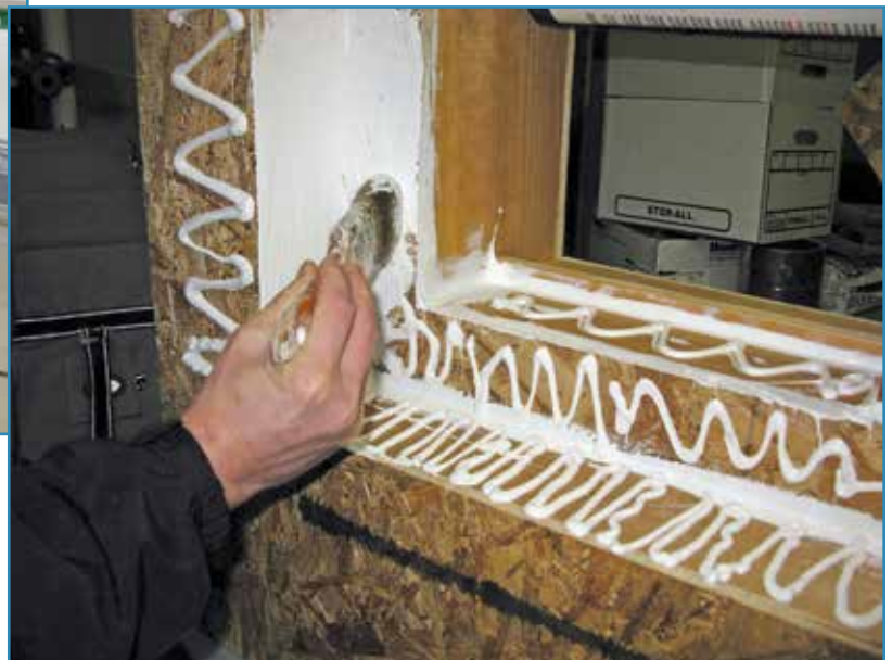
Photo 5 – Fluid-applied WRBs and flashings may be brushed.
