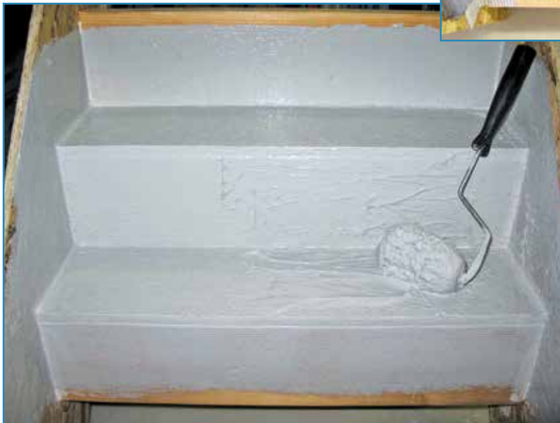
Photo 18 – Full coats may be glopped and rolled to achieve mil thickness.
