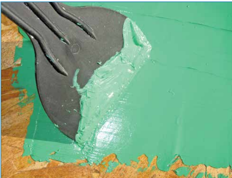
Photo 7 - Silyl-terminated polymer (STP) flashing being troweled.
