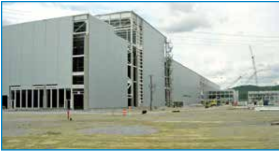
Figure 6 – A siphonic roof drain system was installed on this new Volkswagen plant in Chattanooga, Tennessee. Siphonic design software provided sizing calculations so the installed system would work as engineered. The project scope was more than 46,451 m 2 (500,000 sq. ft.) and included 85 siphonic roof drains.
