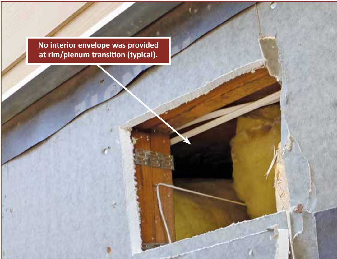
Photo 4 – Perpendicular wall (siding): Plenum space above drop ceiling terminates at inside face of the exterior gypsum sheathing behind the wood board bellyband and the fiber-cement siding.
