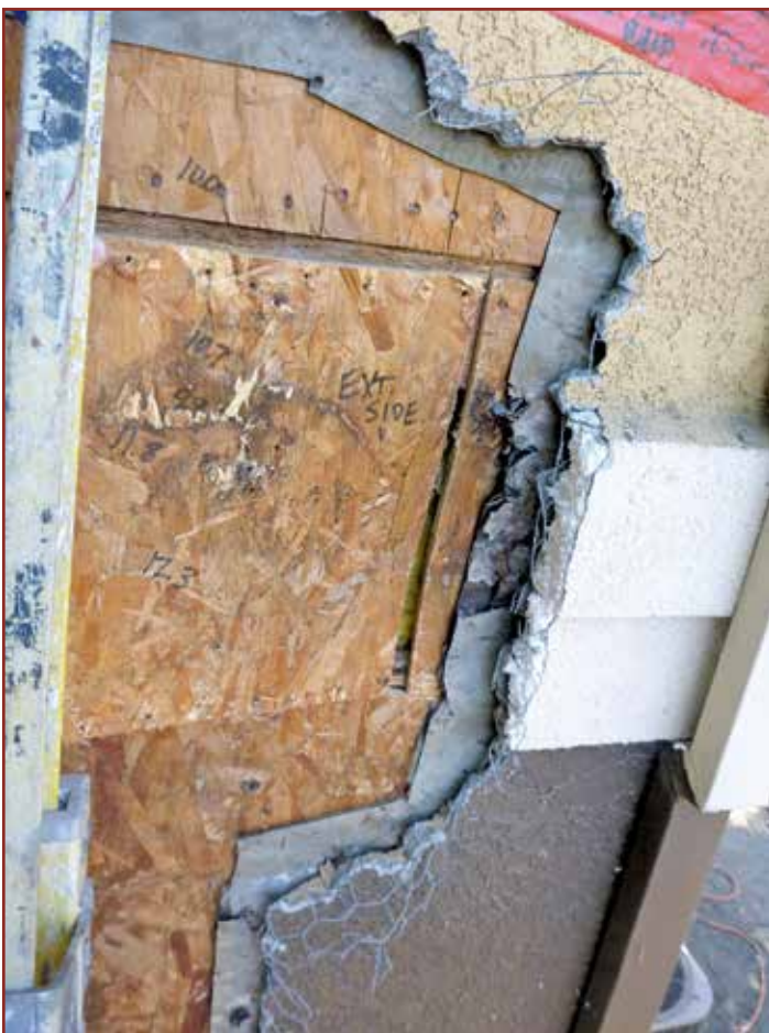
Photo 4 – Perpendicular wall (siding): Plenum space above drop ceiling terminates at inside face of the exterior gypsum sheathing behind the wood board bellyband and the fiber-cement siding.
