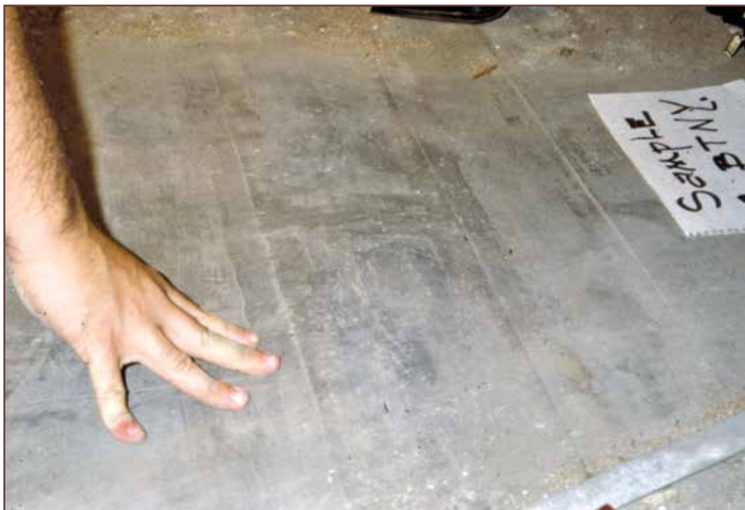
Figure 1 – Tactile testing for moisture.
