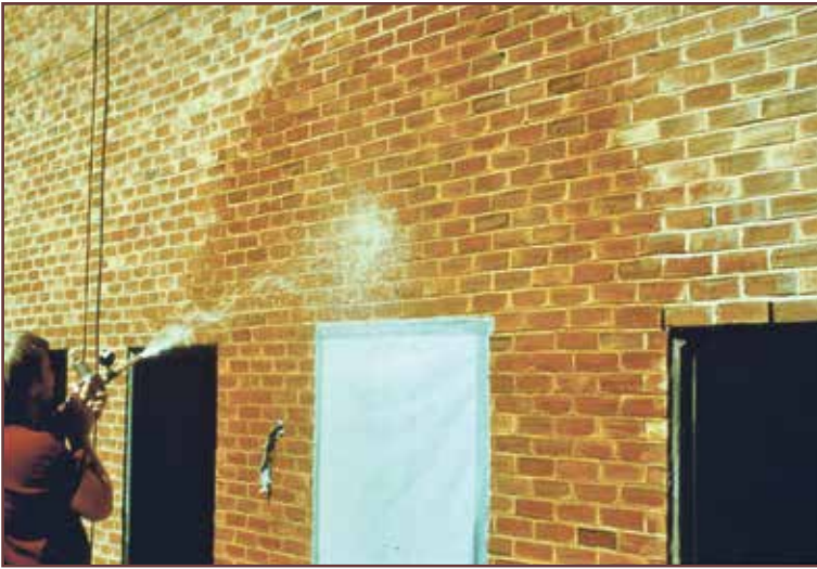
Figure 5 – Poorly executed water testing.
