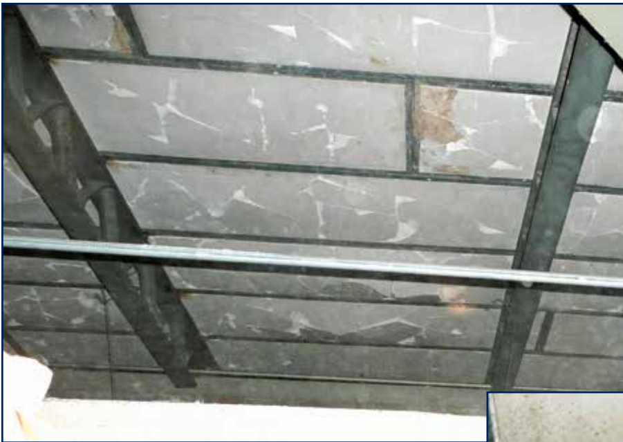
Figure 8 – Example of damage needlessly inflicted on precast lightweight cementitious planks. Contractors working on such a deck should diligently research the proper type and size of fasteners.
