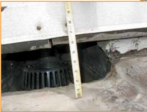
Figure 9 – Roof drain located inside elevation wall.
