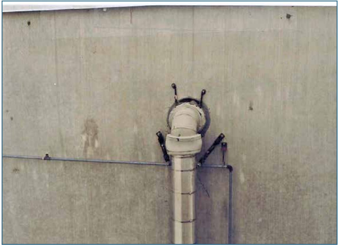
Figure 8 – Insulated refrigeration line penetrating exterior wall of freezer building.
