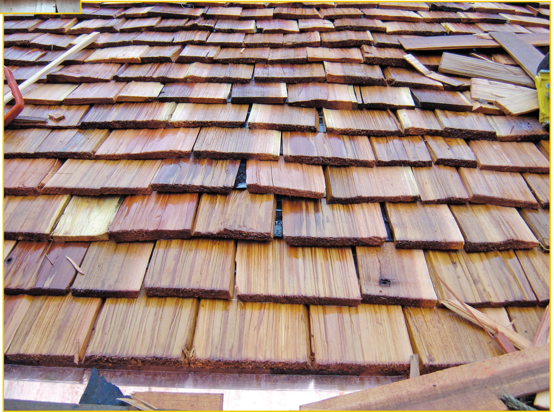
Photo 12 – Rot felting: Ice dam barrier-type product was used for interlayment. Keyway issues and off-grade product are seen here (note excessive flat grain, sapwood, and the knot in near butt end in second course from eave.)
