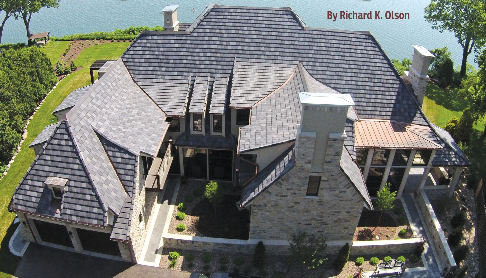
Figure 1 – Concrete flat-tile installation.
