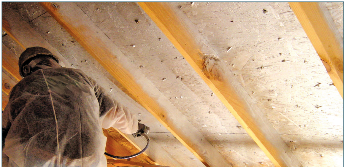
Figure 1 – IRCC installation sprayed to the underside of the roof deck.
