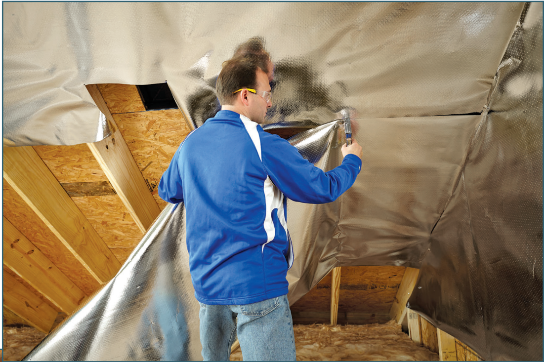
Figure 3 – Radiant barrier installation attached to the underside of the rafter.
