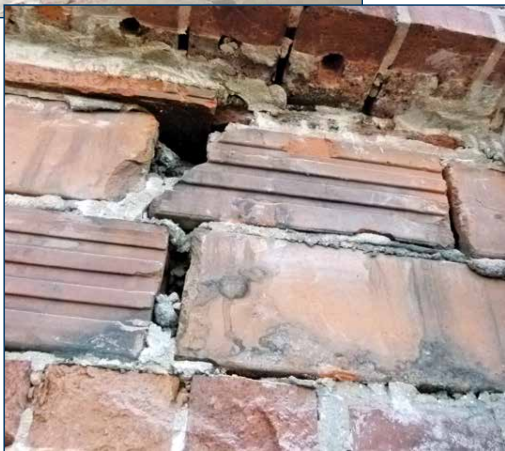
Photo 4 – Use of hollow clay tile units as backup wythes reduces the mass of masonry that can absorb and retain moisture.
