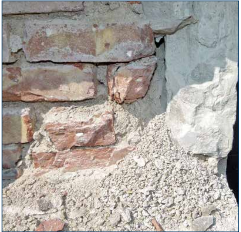
Photo 5 – Deterioration of masonry and mortar within the exterior wall.
