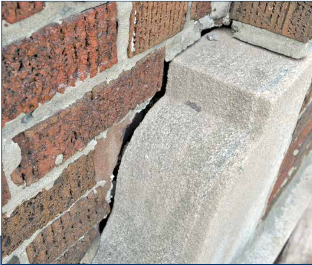
Photo 1 – Open mortar joint between limestone and brick masonry provides a path for water penetration beyond the exterior wythe of masonry.
