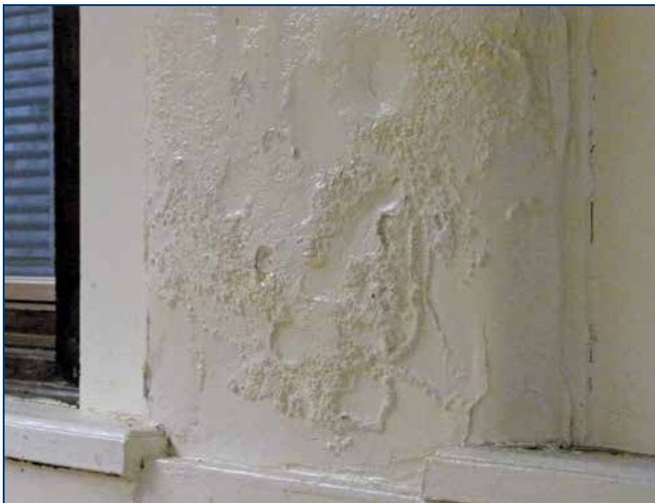
Photo 6 – Deterioration of interior gypsum-based plaster finishes.
