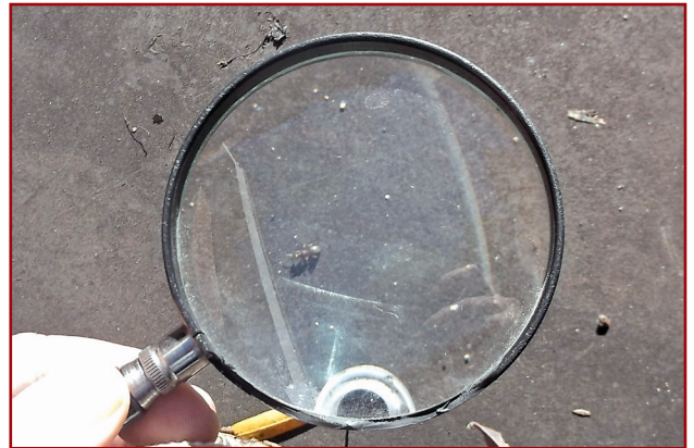
Figure 9 – These creatures were found in abundance on the most recent study carried out by the author. Still, attack from the underside is equally probable. Ants are frequently accused, but other insects may have a similar appetite for rubber membranes.
