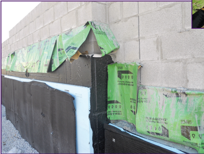
Figure 2 – Sight to be “unseen”—the birthplace of future performance issues with a through-wall flashing (TWF) condition.
