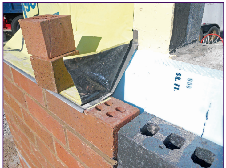
Figure 4 – Full-scale mock-up of a TWF condition on a new construction project. The design intent includes full support for the self-adhering membrane through the wall cavity.
