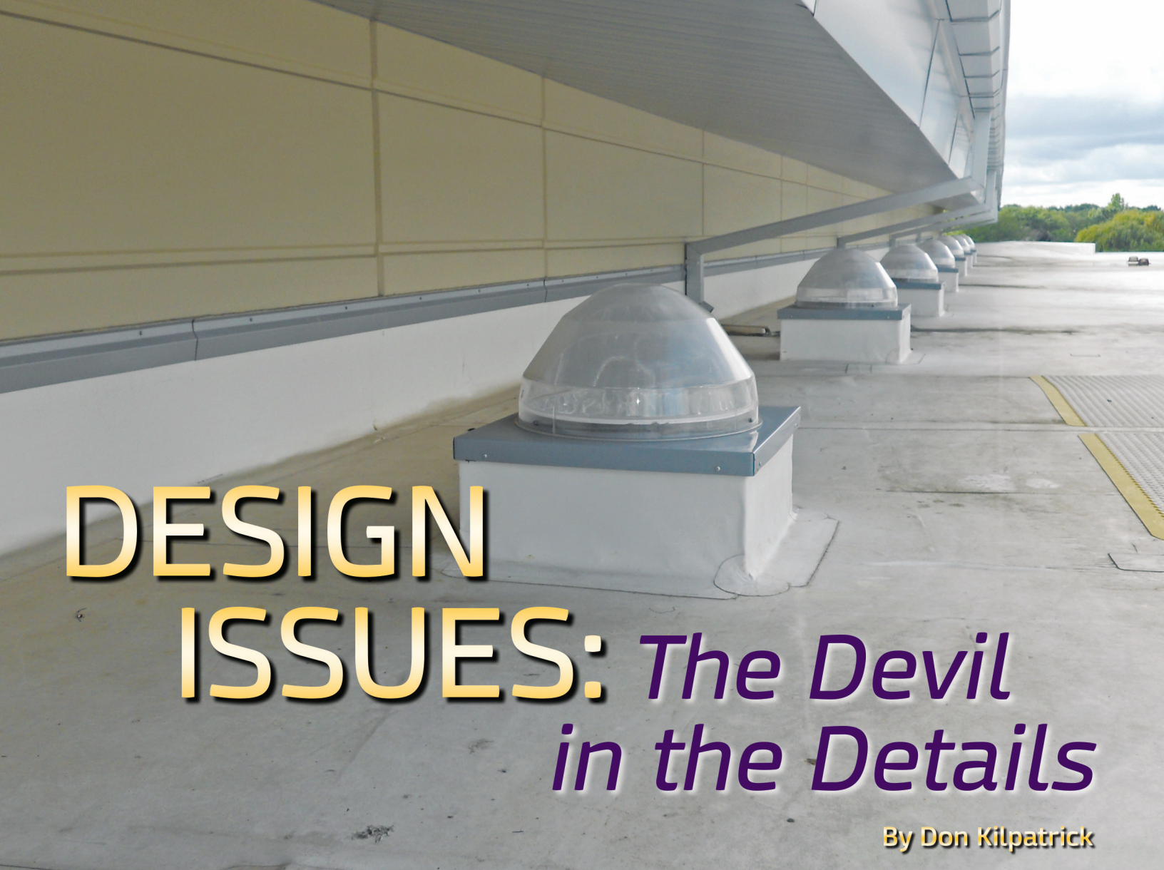
Figure 1— New construction featuring an array of solar tubes. It is assumed that performance could have been optimized if the units were installed without the cover of the overhead-projected soffit.
