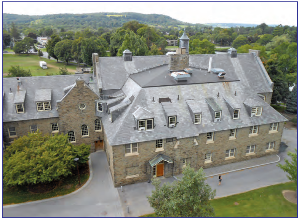
Figure 4 – Prior to 2014 roof replacement project.
