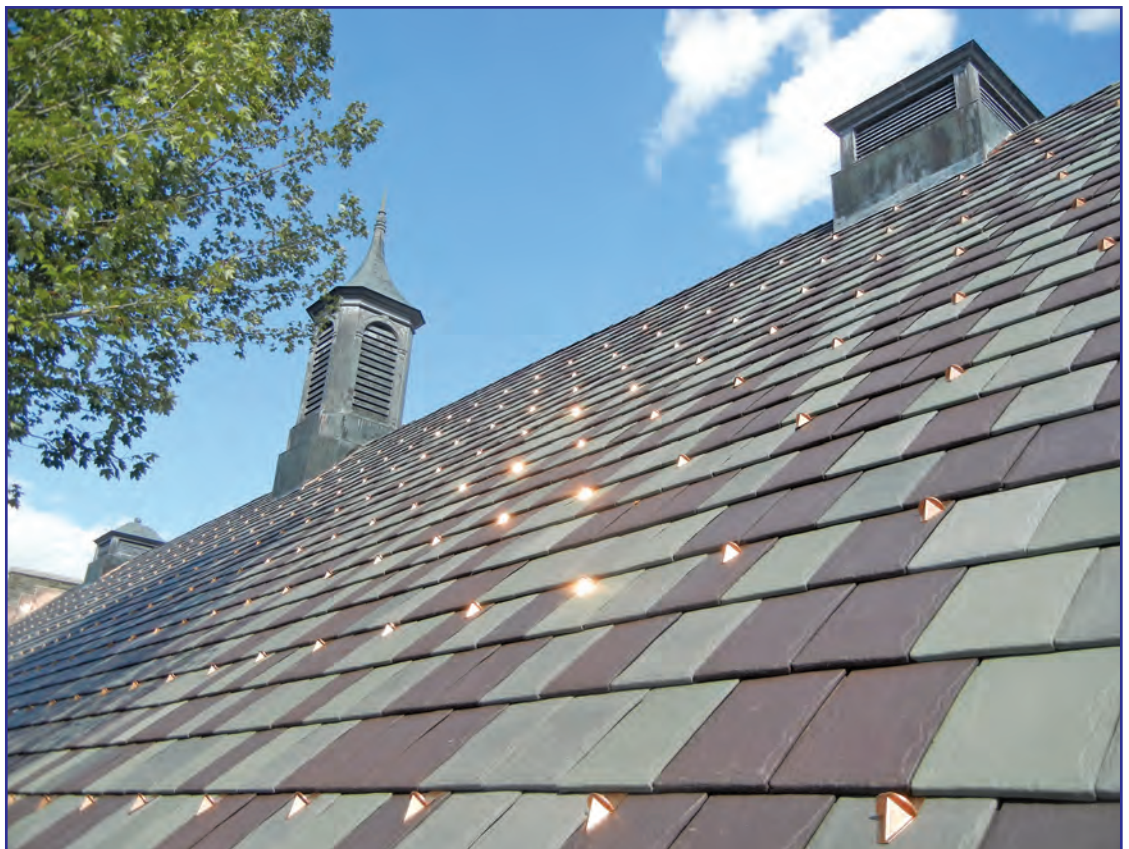
Figure 17 – The completed roof over the dining hall.
