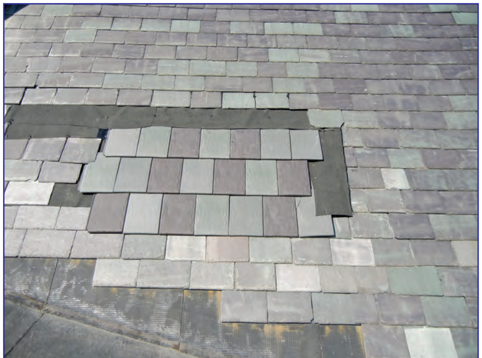
Figure 7 – Clay tile mock-up.
