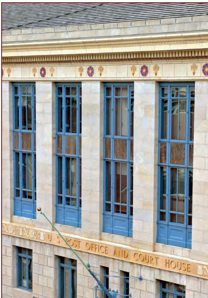
Figure 2 – William J. Nealon Federal Courthouse in Scranton, Pennsylvania.
