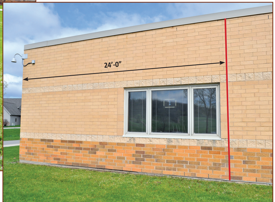
Figure 3A – This veneer expansion joint should have been located on the corner side of the opening. The next closest veneer movement joint to the left of the one shown is 18 ft. around the corner. This makes the expansion joints 42 ft. apart, which is too far, resulting in a crack at the corner of the veneer.
