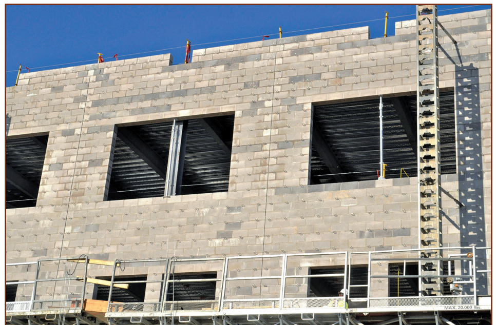
Figure 1 – Control joints properly located between openings.
