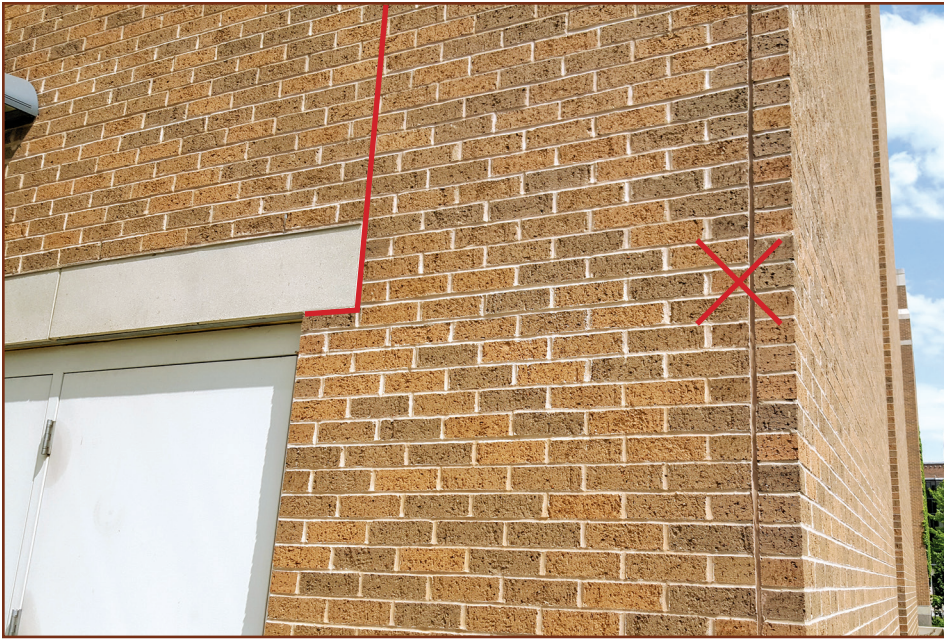
Figure 4 – A veneer movement joint placed 4 in. from the corner will make masonry look panelized. A more functional and aesthetically pleasing solution would be to locate the movement joint at the end of the window lintel, omit the corner movement joint, and then locate a movement joint further away from the corner, not to exceed 20 ft.
