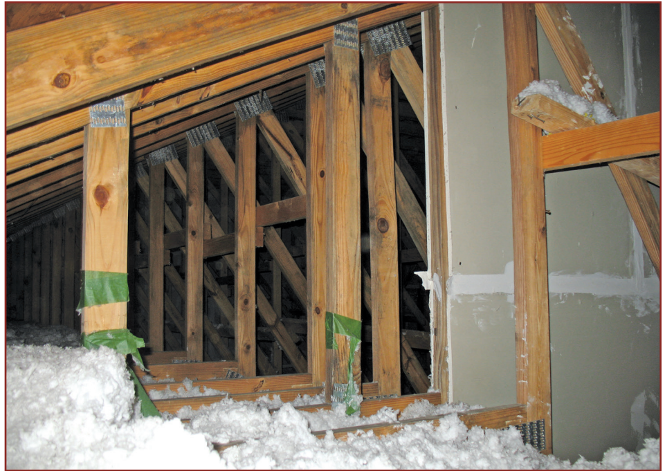
Figure 7 – Incomplete fire-rated wall assembly in an attic.
