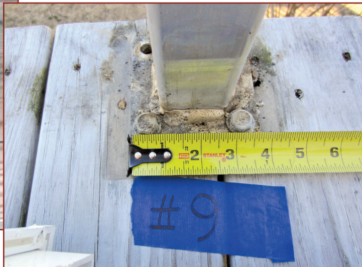
Figures 5 and 6 – Inadequate guardrail attachment.
