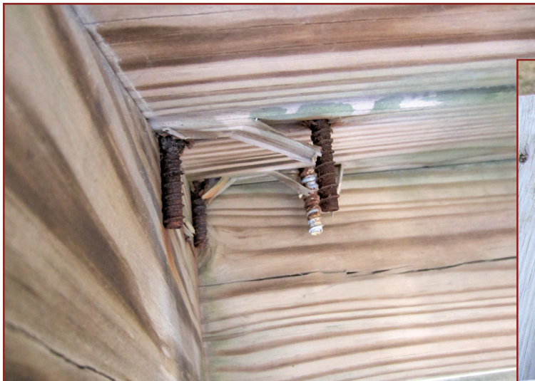
Figures 5 and 6 – Inadequate guardrail attachment.
