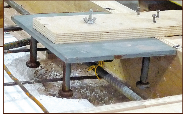
Figures 3A and 3B – Voids in the insulation foam board (3A) are made to accommodate steel embeds (3B) that are needed to connect the panel to the structure of the building. Depending on the thickness of the insulation, the void may span part of or the entire depth of the insulation board.
