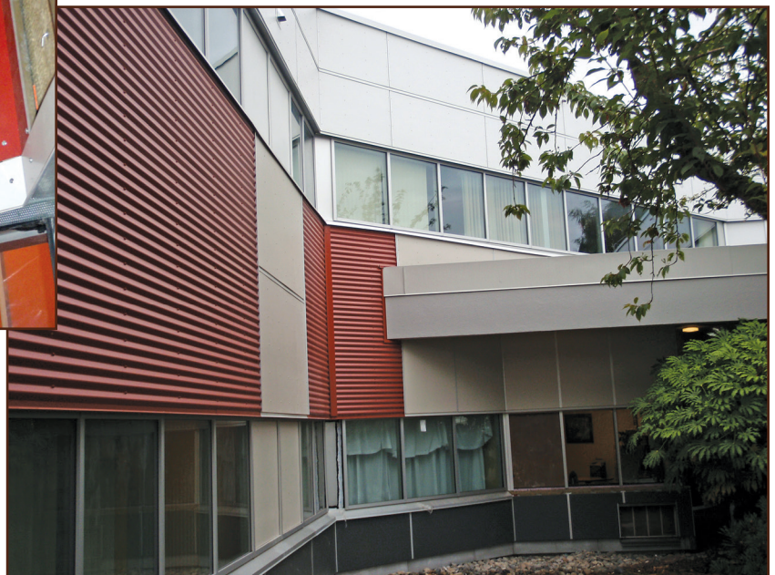
Figure 5 – The new wall claddings after completion of Case Study One.
