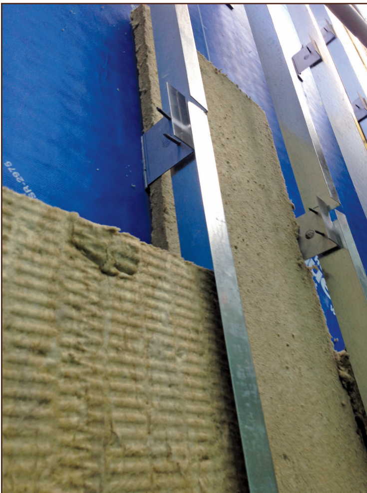
Figures 7 – Clip used in Case Study Three with aerogel insulation.
