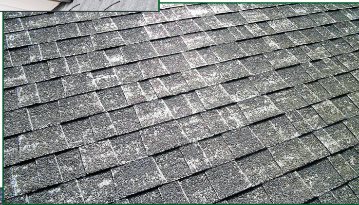
Figures 5A, 5B, and 5C – Attempting to repair these shingles would be futile. Yet it would be inaccurate to characterize them as brittle. They are instead highly weathered, impractical to repair, and should be in a landfill.
