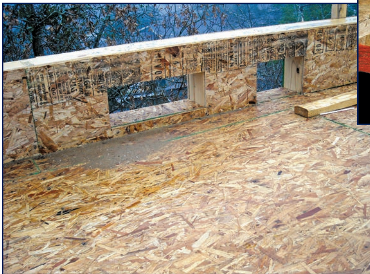
Figure 1 – Consultants are likely to encounter OSB in both pitched and low-slope assemblies. Here, a quite large facility used OSB for the roof deck, the inboard face of parapets, penthouse cladding, and elsewhere.
