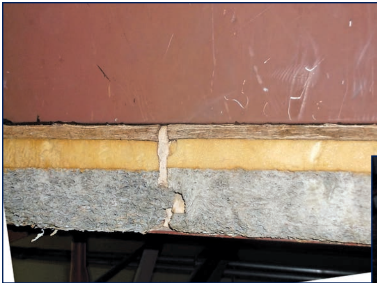
Figure 4 – OSB can be integrated with structural cement fiber planks along with isocyanurate foam as the core. Here, fire-safing material was applied at joints.
