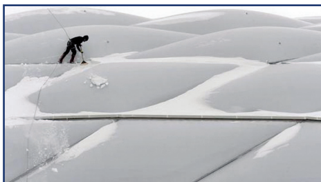
Figure 9 – Manual removal of snow from an ETFE system. Photo credit: SurfaceDesign.
