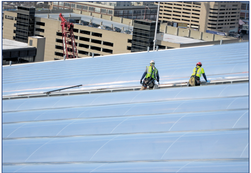
Figure 20 – Installation of ETFE cushions.
