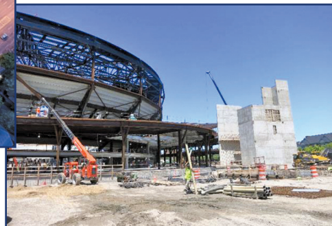
Figure 25 – Current construction of arena and surrounding structures.
