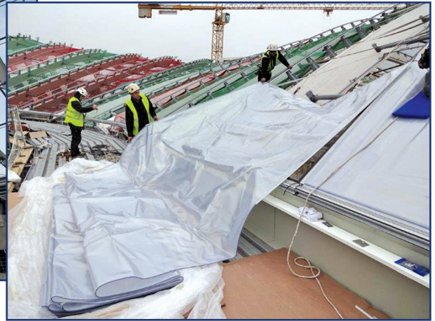
Figure 15 – Installation of ETFE cushion. Photo by Birdair.
