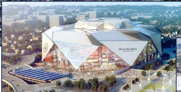
Figure 22 – Rendering of the Mercedes Benz Stadium showing ETFE roof system and ETFE cladding system. Photo by HOK.
