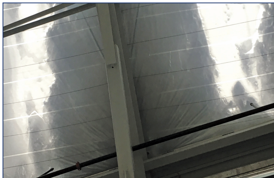
Figure 10 – An ETFE system in a deflated state, supported by snow cables, with snow load. Photo by SurfaceDesign.
