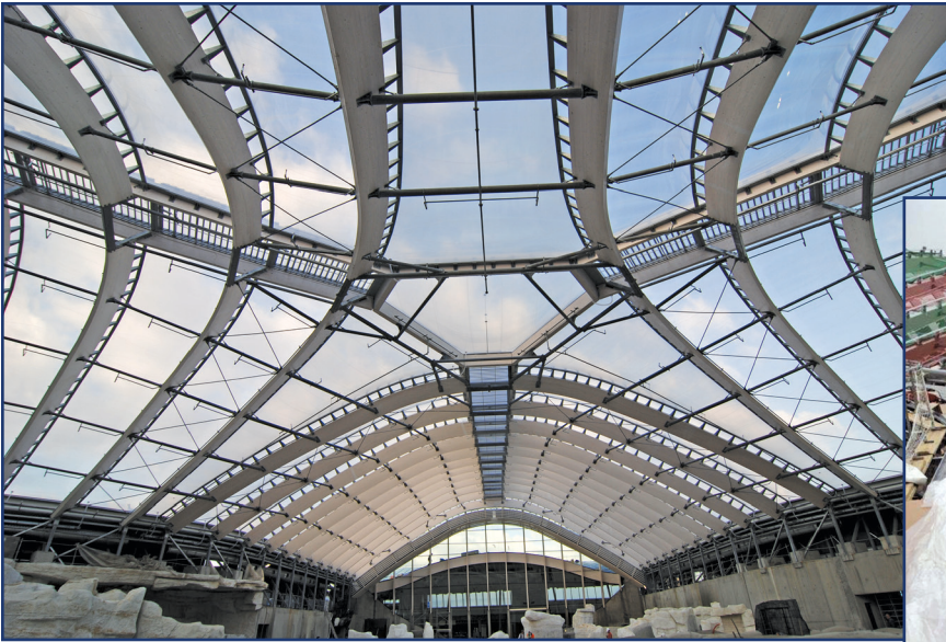
Figure 16 – ETFE roof system from interior. Photo by Birdair.
