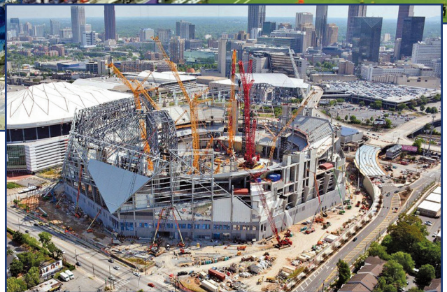
Figure 23 – Current construction of stadium. Photo by www.11Alive.com .
