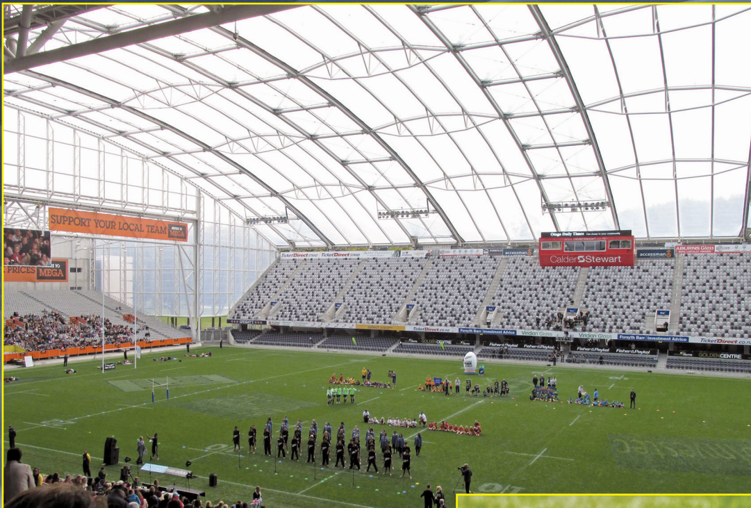
Figure 11 – ETFE roof spanning the playing field.
