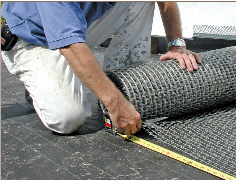
Figure 1 – Nonmetallic plaster bases cut easily.
