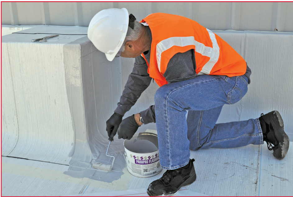
Figure 5 – Fully reinforced, seamless PMMA flashing applications effectively address both standard and challenging details.
