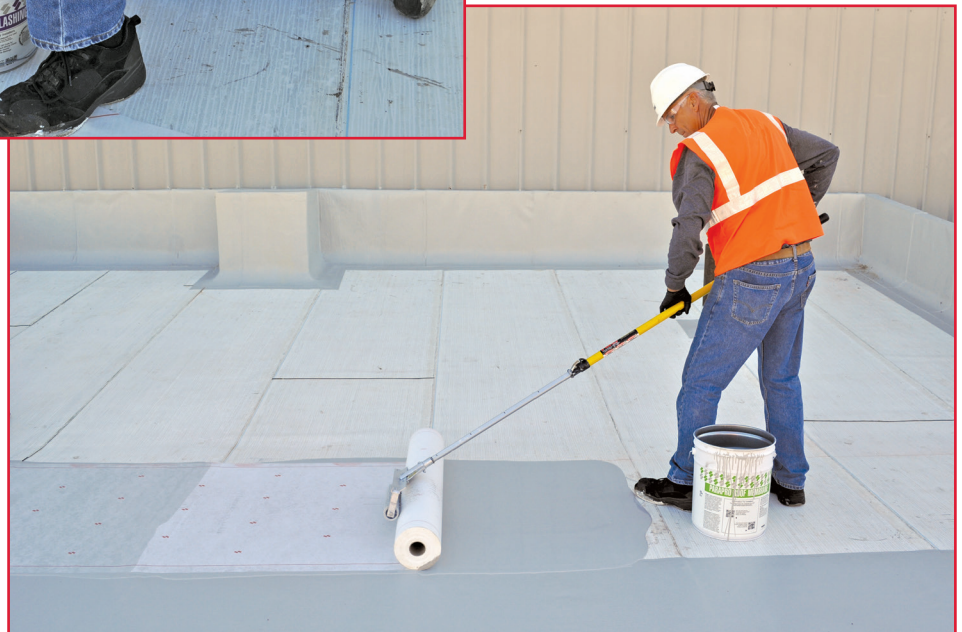
Figure 6 – PMMA roof membrane systems are fully reinforced, layered applications consisting of one coat of primer (if required) and a waterproofing membrane comprised of two resin waterproofing coats and polyester fleece fabric.
