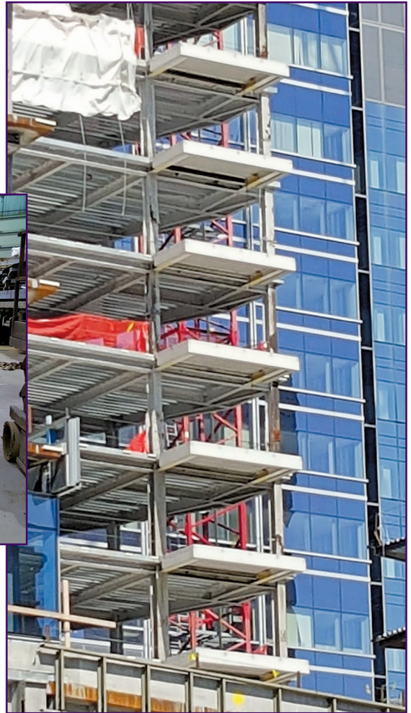
Figure 7 – Precast balconies placed directly on AFC-coated outriggers.
