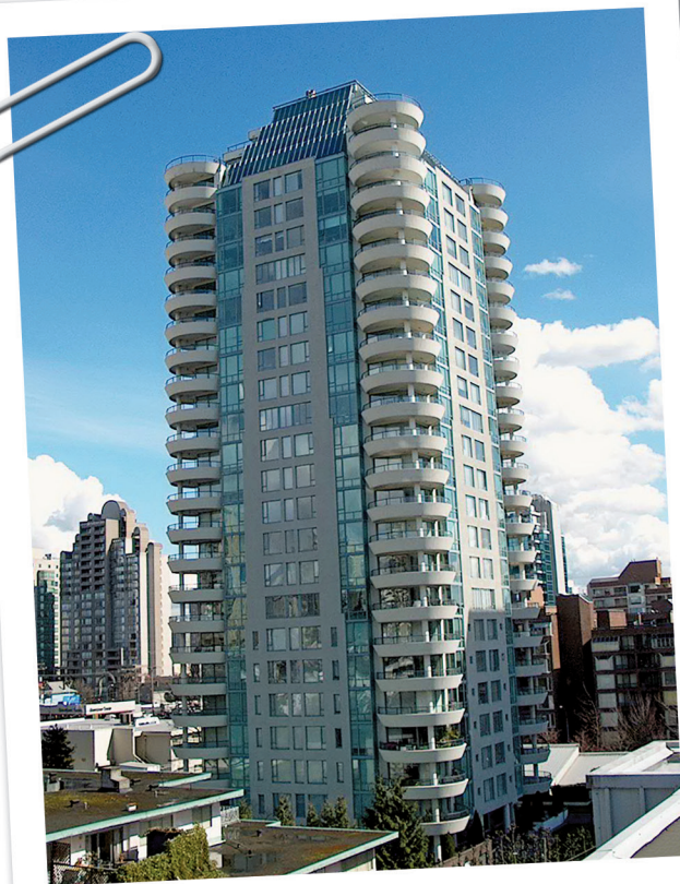
Figure 1 – View of building as originally constructed.
