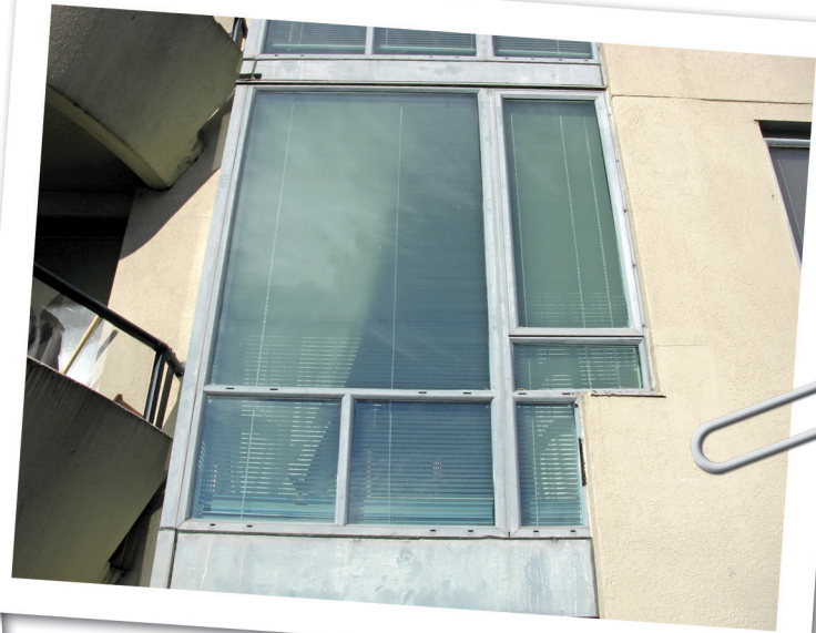
Figure 4 – Typical window assembly set into EIFS cladding; as built, there was no drainage from behind the spandrel panels.
