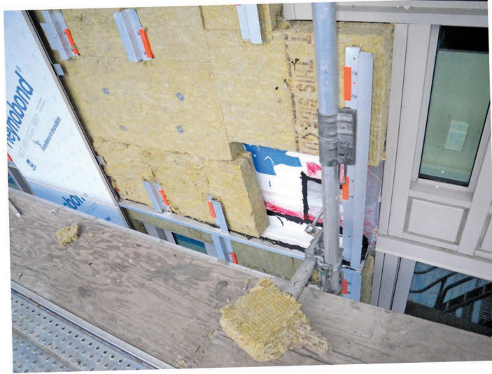
Figure 6 – Wall assembly under construction.
