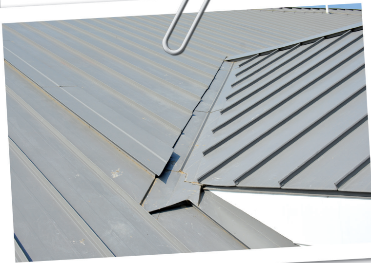
Figure 10 – Completed expansion joint/valley intersection (north side).
