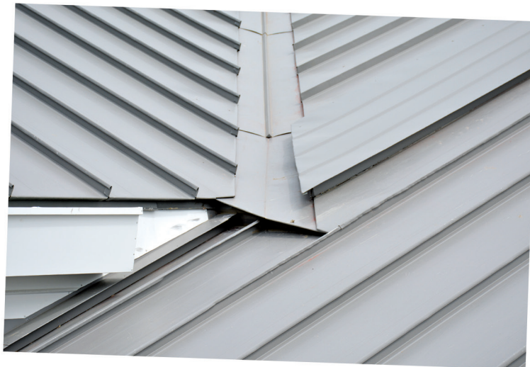
Figure 11 – Completed expansion joint/valley intersection (south side).
