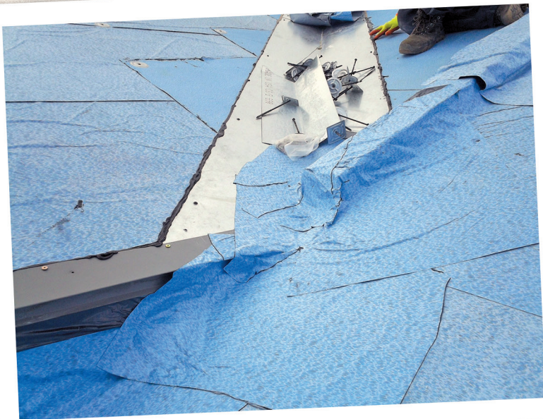
Figure 5 – Expansion joint valley intersection prior to panel and flashing installation.
