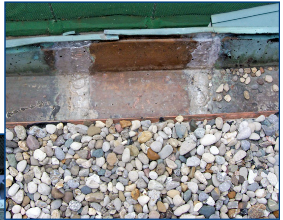
Figure 4 – Completed proper repair of copper gutter.
