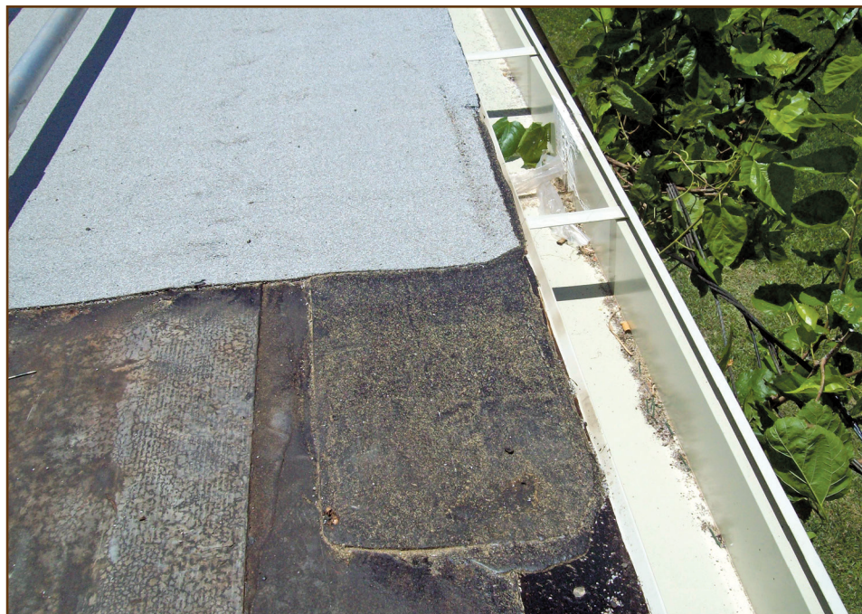
Figure 4 – Metal edge, strip-in, and cap sheet.
