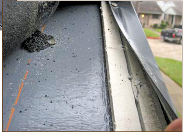
Figure 19 – Fasteners for rake flashing installed in joint between fascia cement boards.
