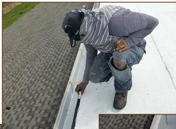
Figure 6 – Tooling sealant.
