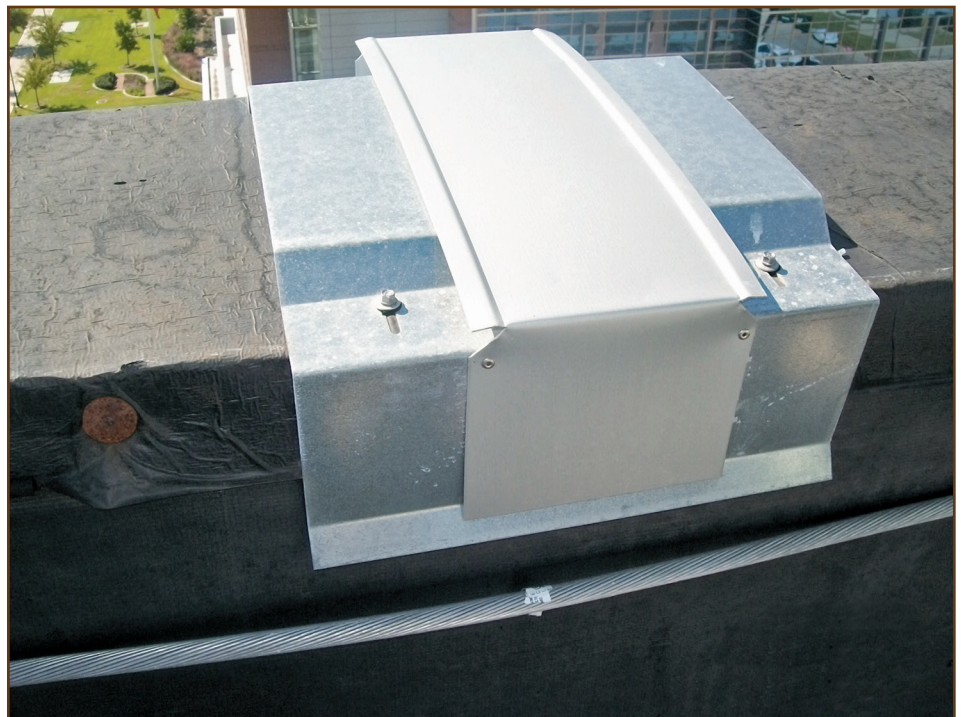
Figure 17 – Typical cleat/chair for coping.
