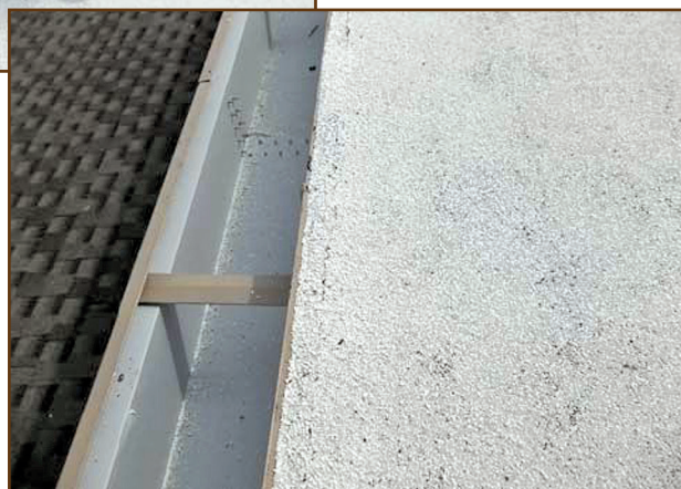
Figure 7 – Granules embedded in sealant.
