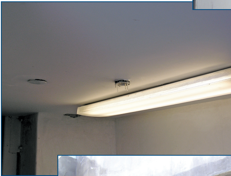
Figure 12 - Water leaking through residence utilities. Note the formation of stalactites from chronic leakage. The swimming pool is directly above this finished living space.
