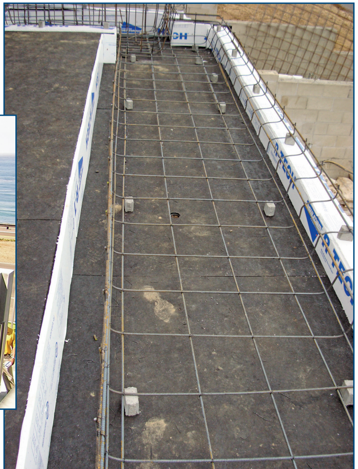
Figure 9 – Geotextile drainage composite laid flat.
