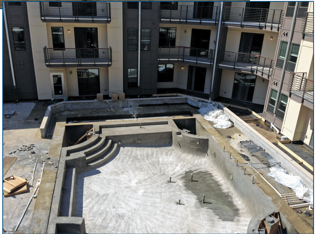
Figure 15 – Overview of pool during construction.
