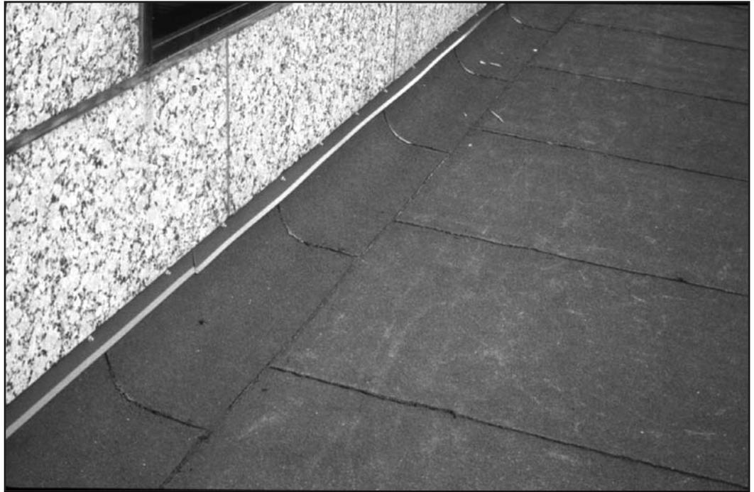
*This building has a glass-reinforced base sheet SBS with a glass-reinforced polyester SBS FR cap, applied with a cold adhesive by squeegee from five-gallon pails.*
