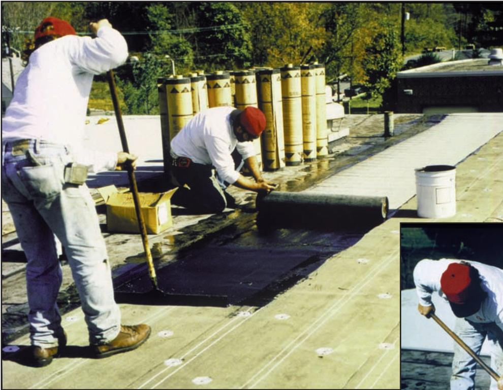
*Workers install an SBS cap sheet and polyester-reinforced SBS smooth membrane with modified bitumen cold adhesive over an MB base sheet. Seams are heat-welded.*
