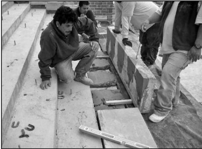
One major drawback to concrete stairs is if the system requires repair, the removal of concrete is time consuming and expensive.
