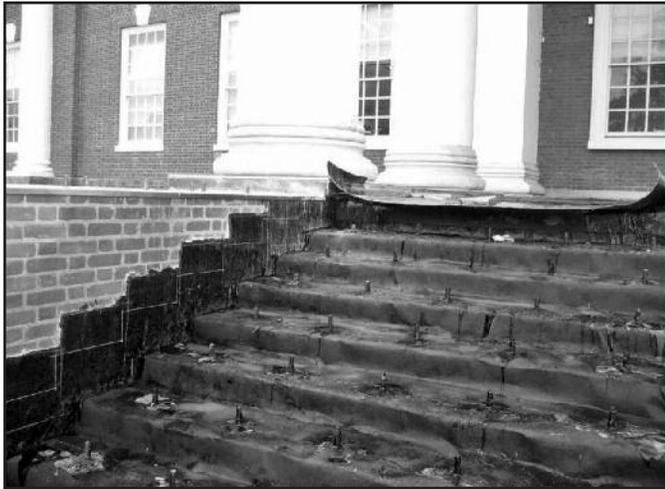
prior to installing drainage layer, insulation, filter fabric, and overburden components to locate and address any leaks. Leaks are much easier to address before the membrane is covered with overburden, which requires significant effort to remove in order to access and repair the membrane. Common water-testing strategies include standing-water and spray-rack tests.
