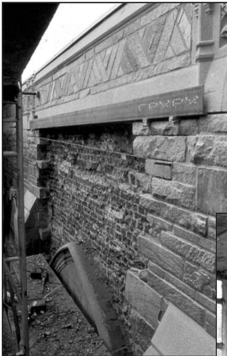
**Figure 1 – View of stone masonry removal during a rehabilitation project to allow for the installation of dedicated waterproofing above window openings in an historic mass masonry wall.**
