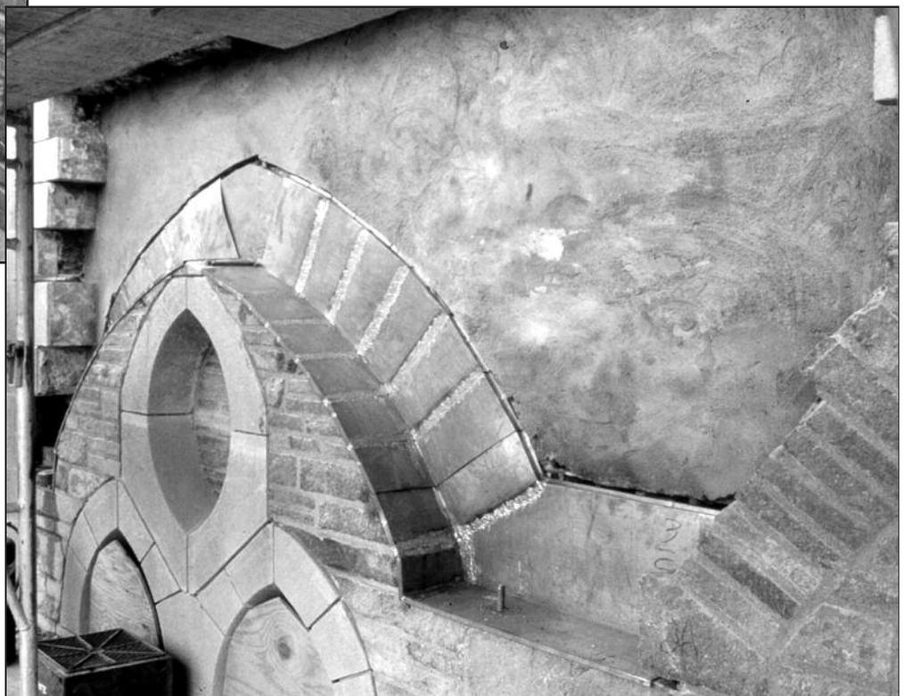
**Figure 2 – View of dedicated waterproofing and flashing installation in an historic mass masonry wall assembly during a rehabilitation project.**
