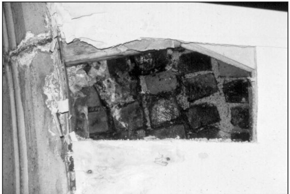
**Figure 7 – View of moisture accumulation and masonry damage on the interior face of an historic masonry-wall system following the installation of extruded polystyrene (XPS) insulation behind the interior plaster finishes during a recent rehabilitation project.**
