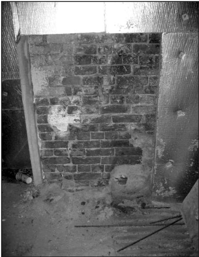
**Figure 6 – View of the interior face of a brick-masonry wall system where deterioration resulted from the installation of a vapor barrier (foil facer) and thermal insulation.**
