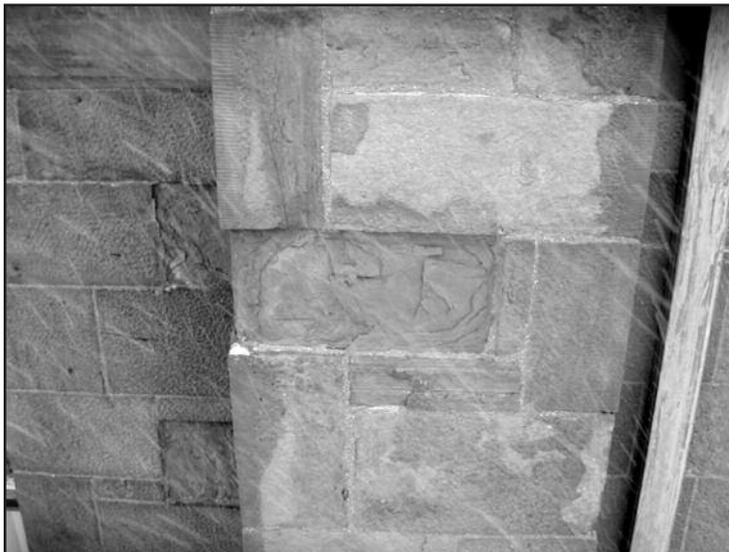
**Figure 4 – View of stone masonry deterioration from freeze-thaw following the installation of thermal insulation on the building interior.**
