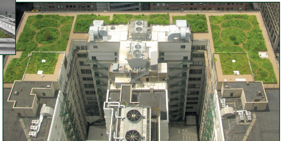
Figure 4 – Green roof on the Chicago City Hall building.
