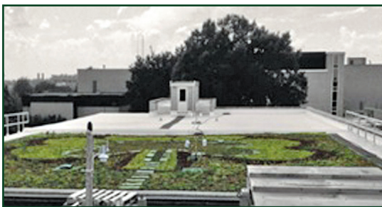
Figure 3 – Green roof on Emerson Electric Company Hall.
