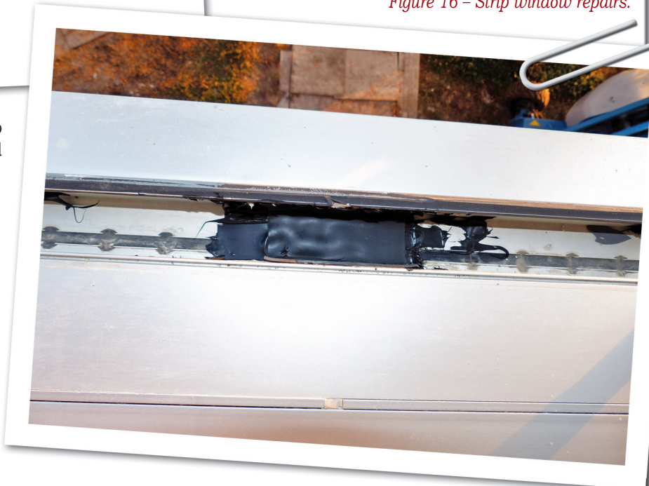
Figure 16 – Strip window repairs.
