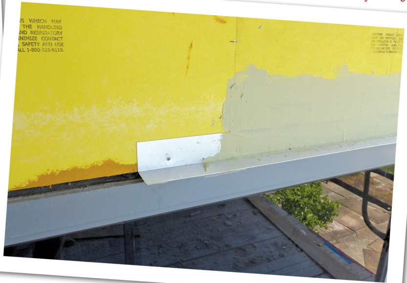
Figure 10 – Window head flashing.
