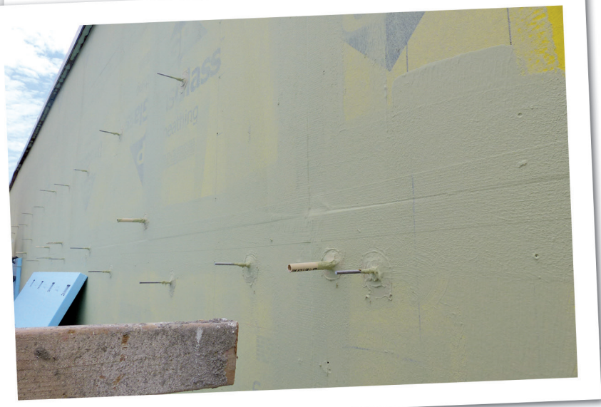
Figure 13 – WRB application around signage support anchors.
