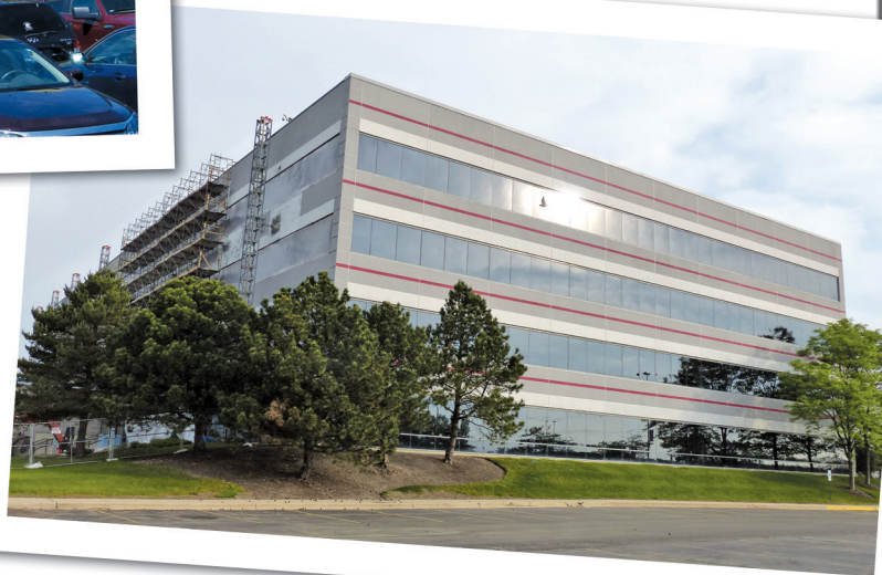
Figure 18 – Completed east elevation.
