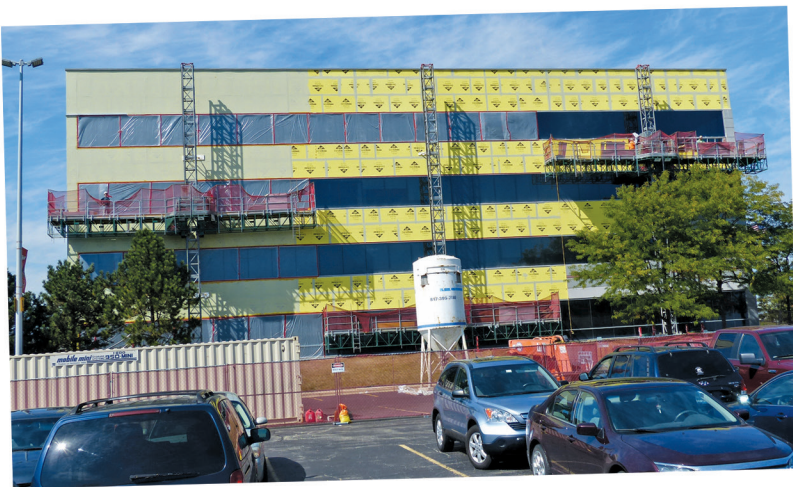
Figure 17 – East elevation during construction.
