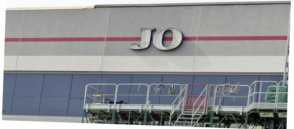
Figure 14 – Reinstallation of signage over finished stucco cladding.
