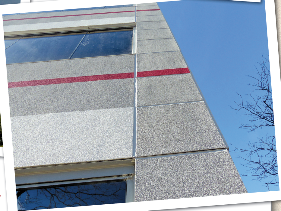
Figure 8 – Stucco system designed to replicate original appearance.
