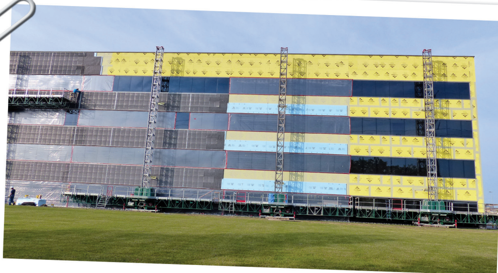
Figure 19 – Metal lath installation several days after sheathing and insulation.
